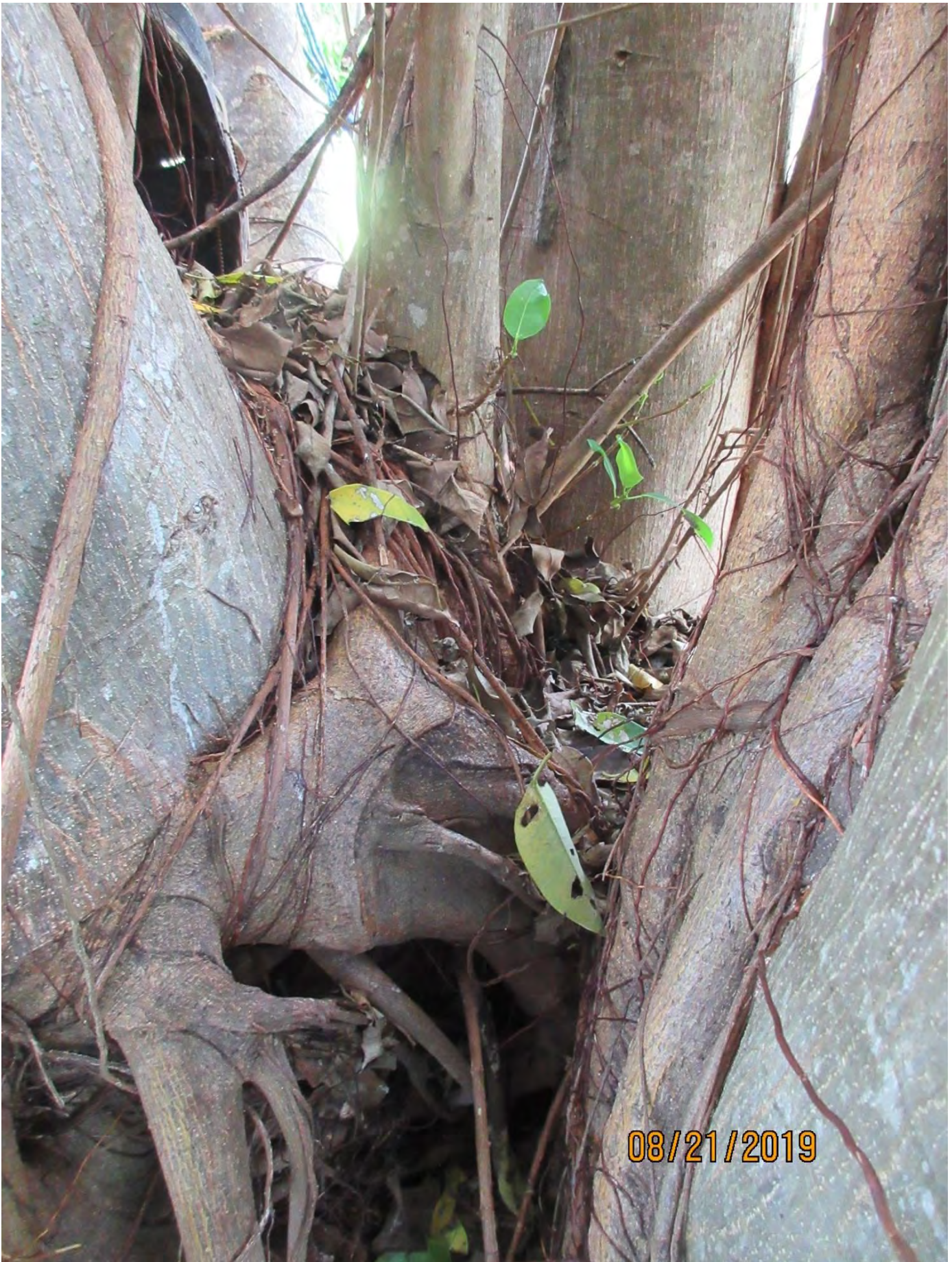
Close up photo of base of tree area view 2.
