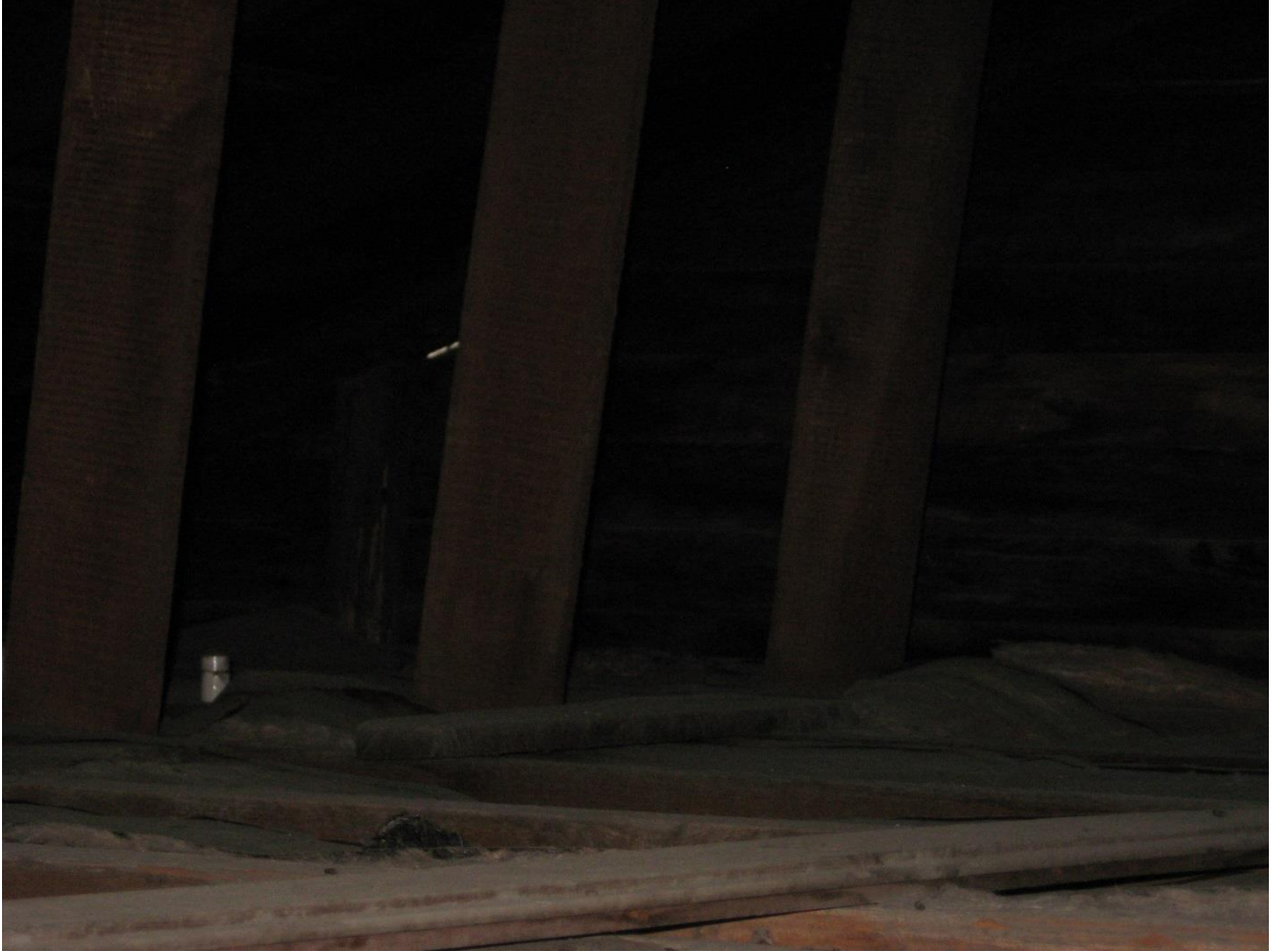
Can see light through the siding in attic
