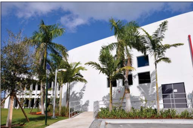
VIEW OF THE BUILDING FROM THE PARKING AREA
