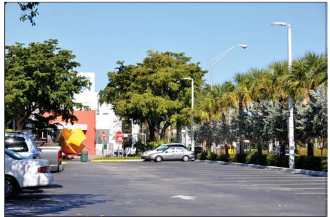
VIEW OF THE MAIN BUILDING ENTRANCE FROM THE PARKING AREA
