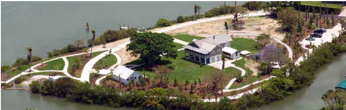
Phase 1 under construction (2011)
