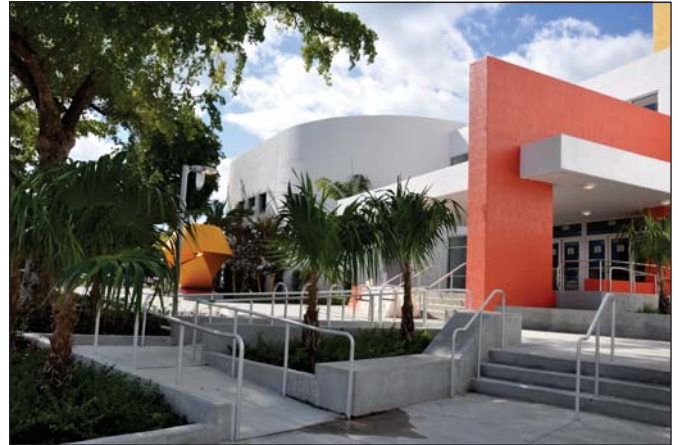
MAIN ENTRANCE COURTYARD AND SCULPTURE
