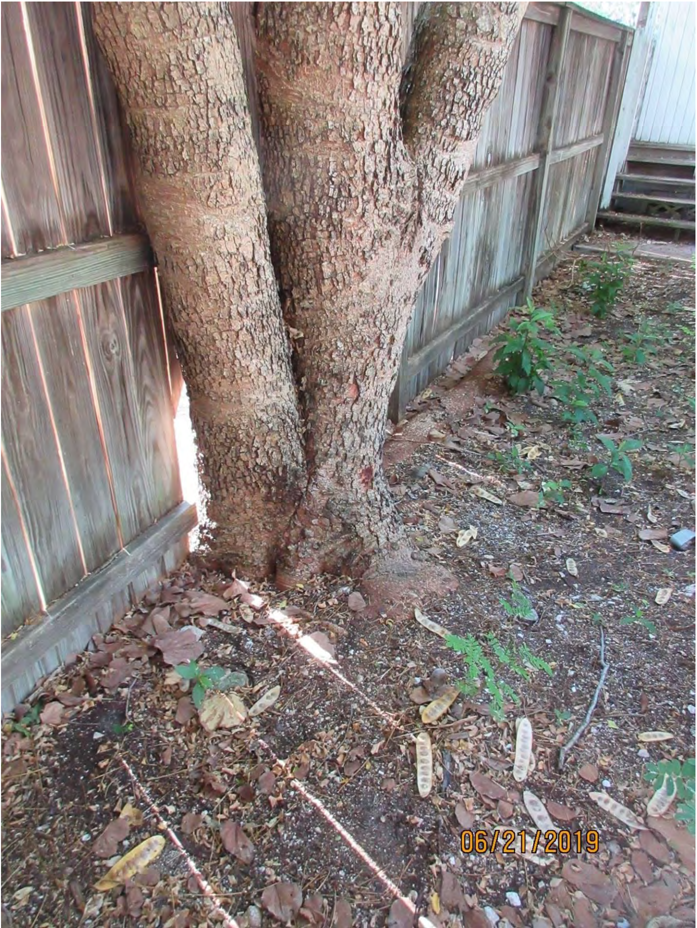
Photo of base of tree, view 1.
