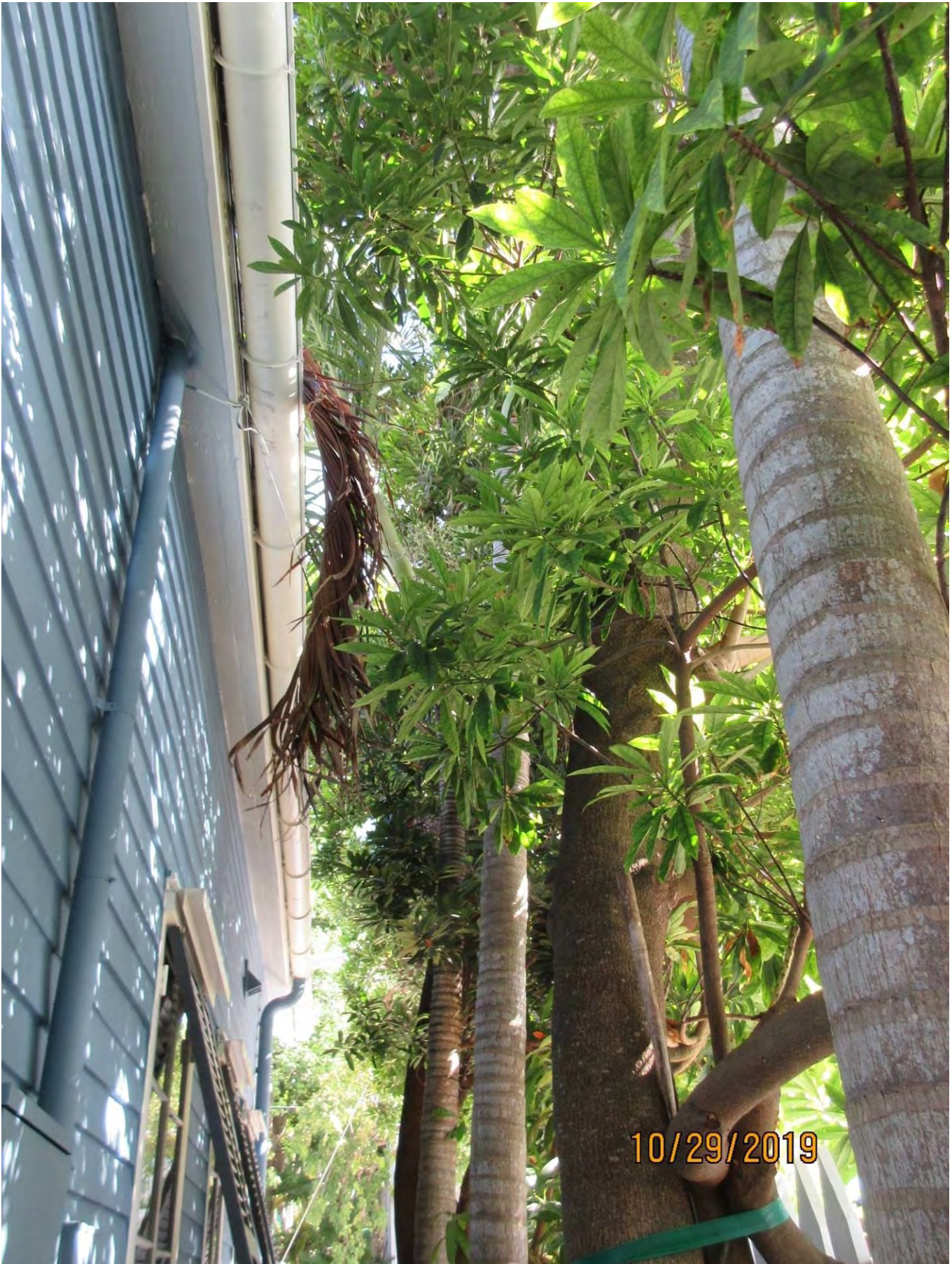
Photo showing the tree canopies in relation to the structure.
