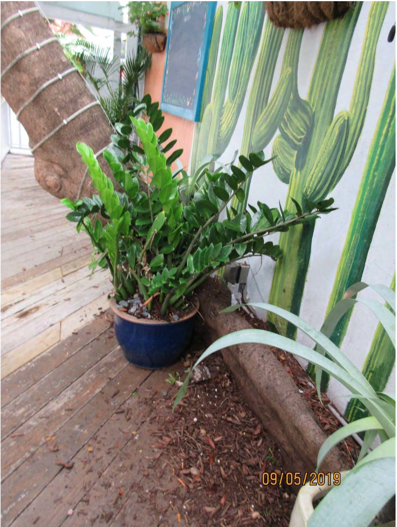
Photo showing base of Royal Poinciana tree against neighboring structure, view 1.
