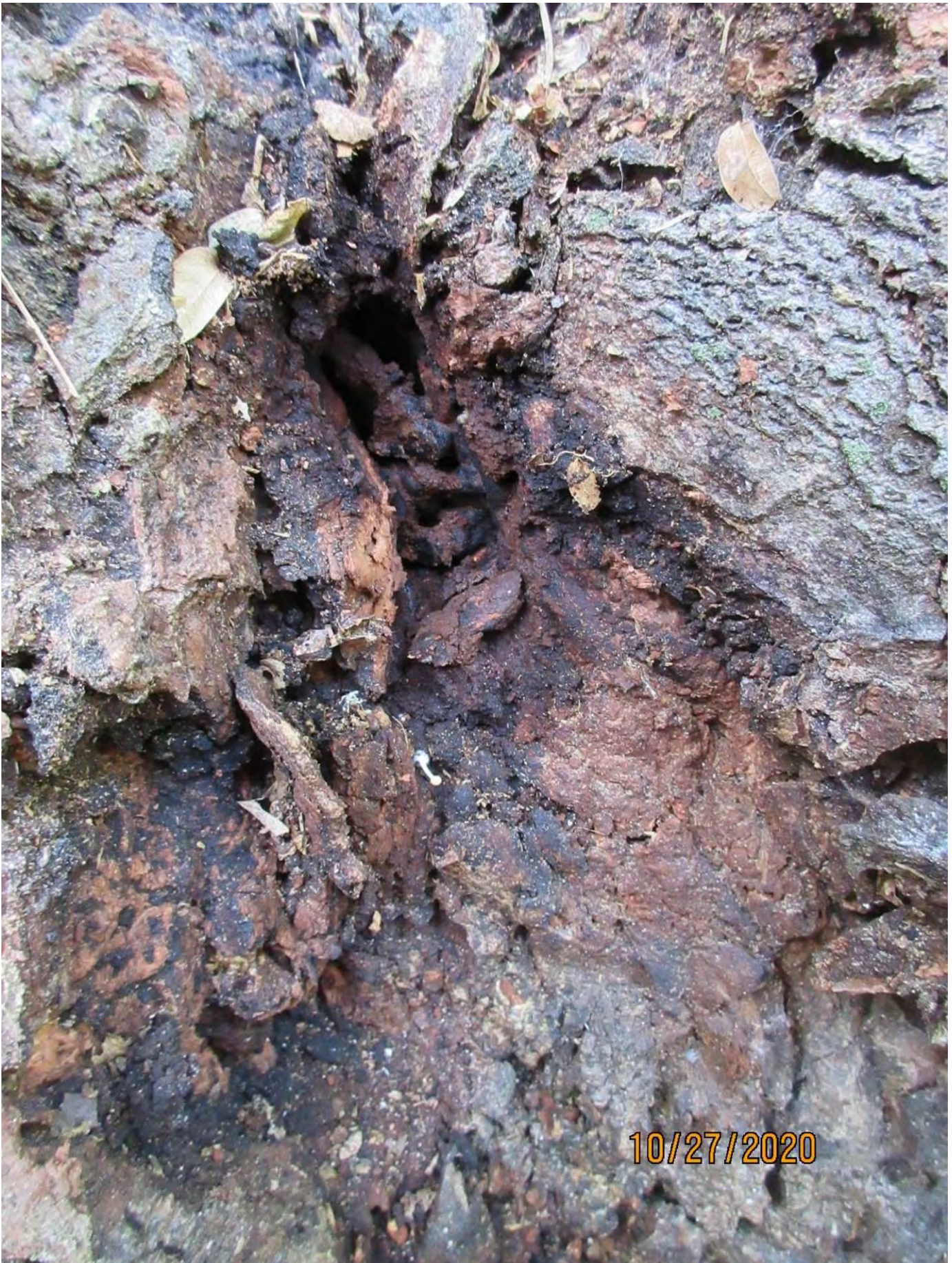
Close up of termites area at base of tree, view 2.
