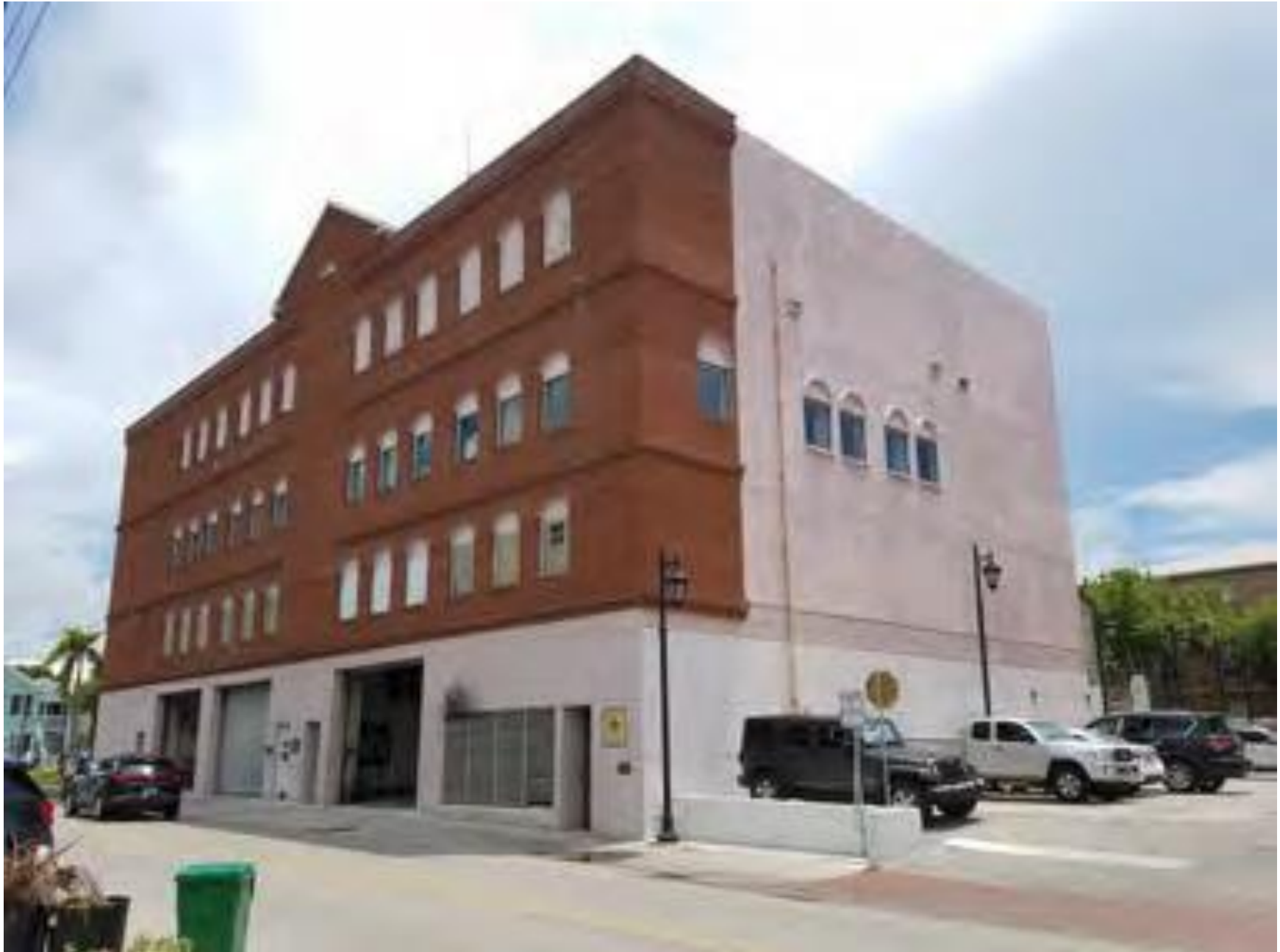
521 Thomas Street, Key west, Florida 33040 SITE VISIT
