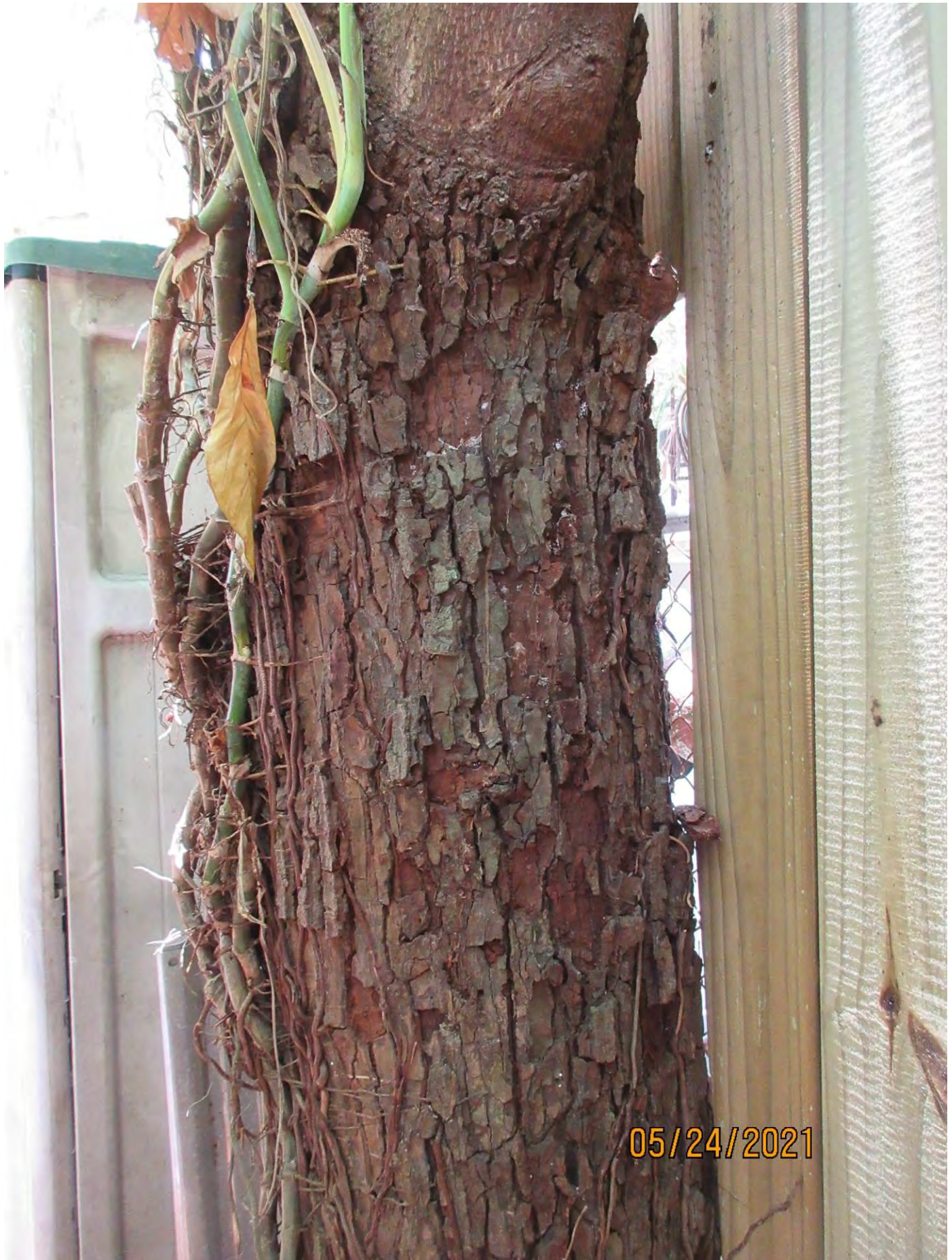
Photo of tree trunk and completed fence, view 5.
