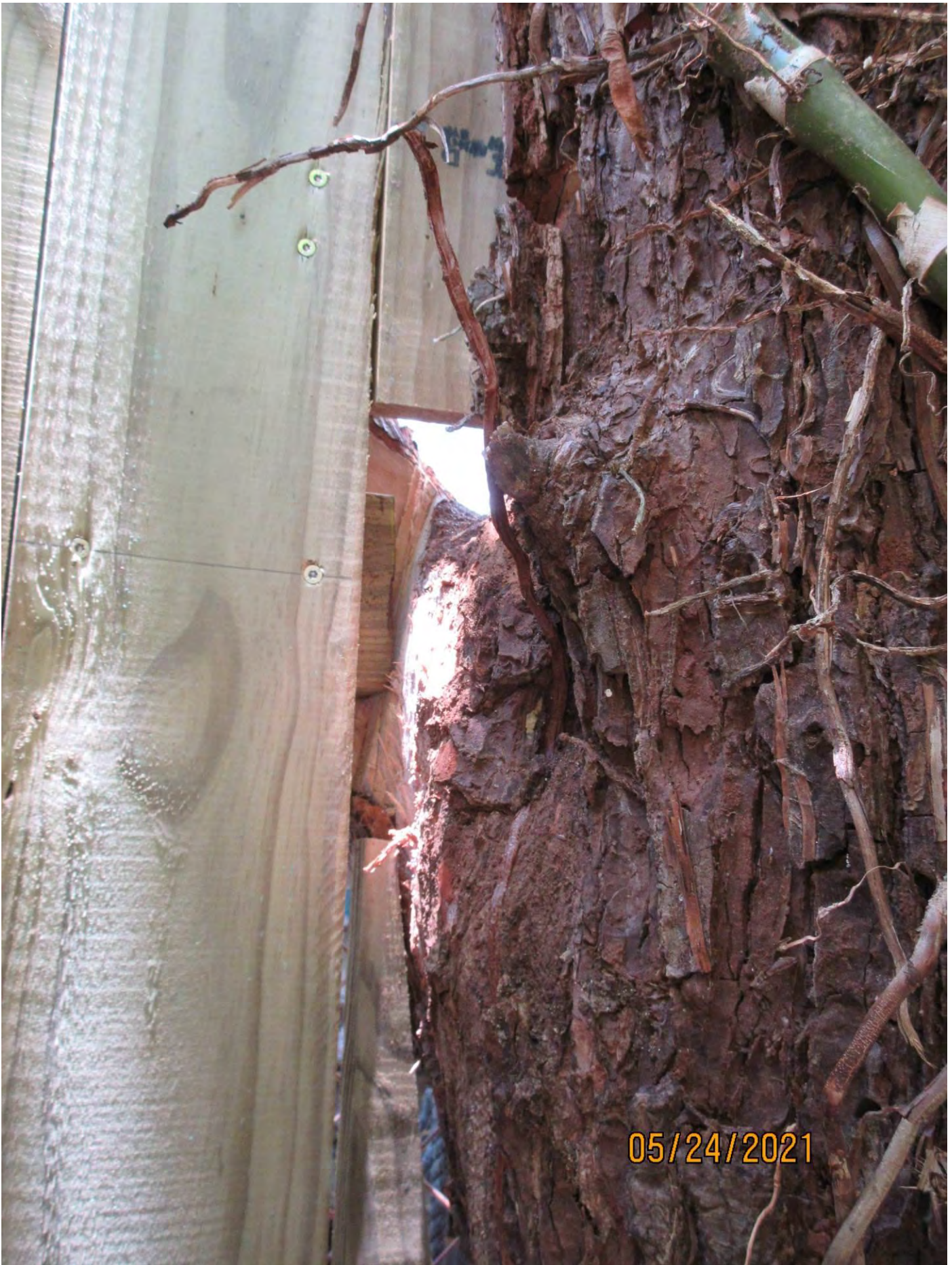
Photo of tree trunk and completed fence, view 2.
