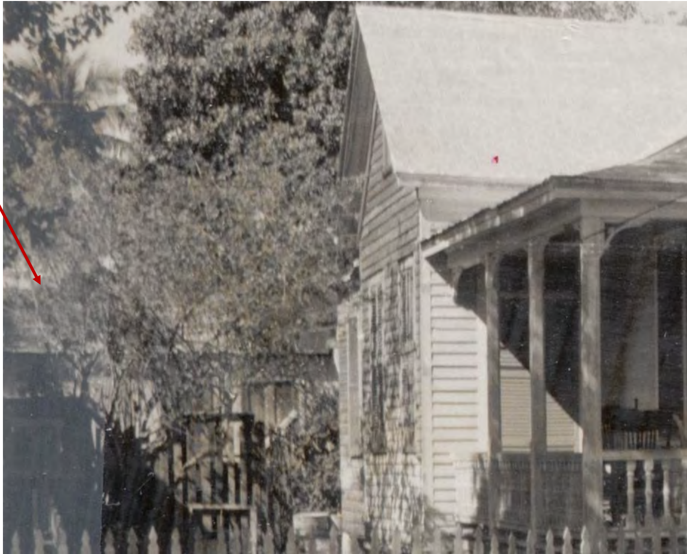
Detail of the rear structure behind the principal house from circa 1965 photograph. The one-story structure has a side gable roof.
