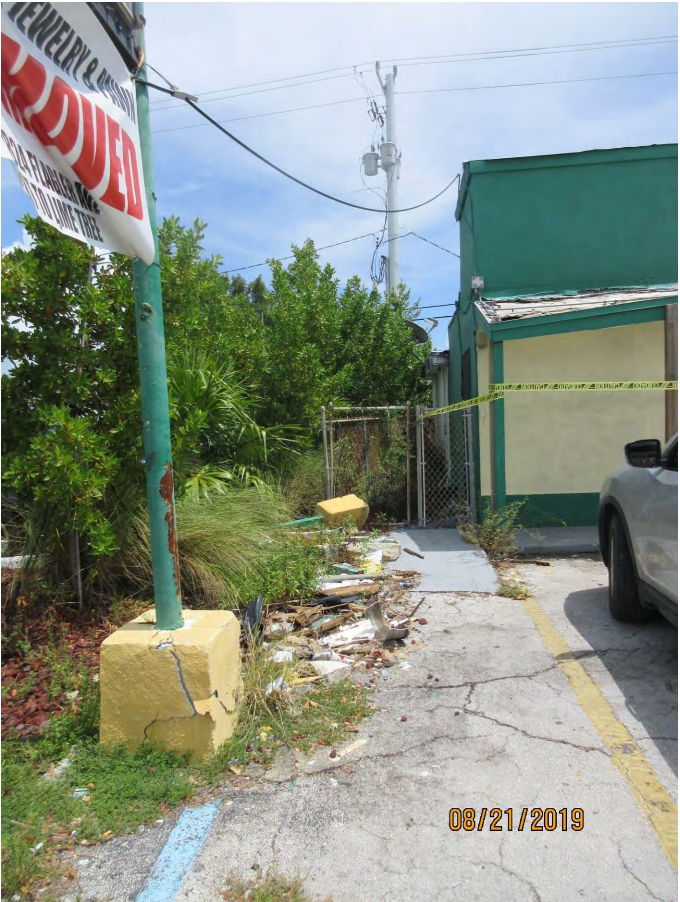
Photo looking south down the eastern property line view 1.
