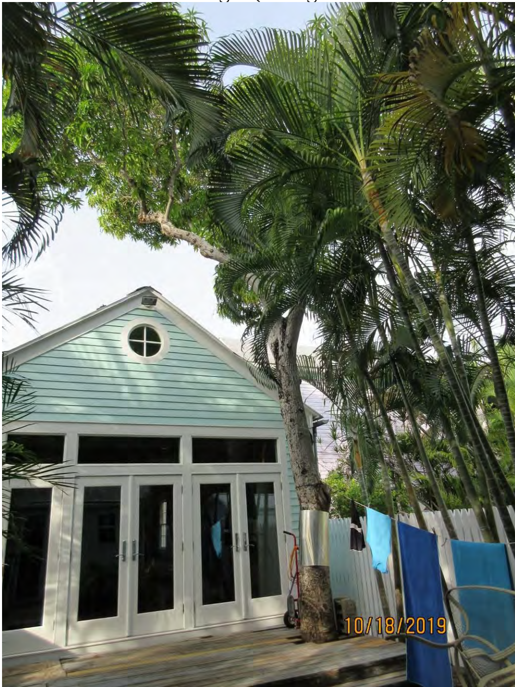
Photo of mango tree in back yard near structure
