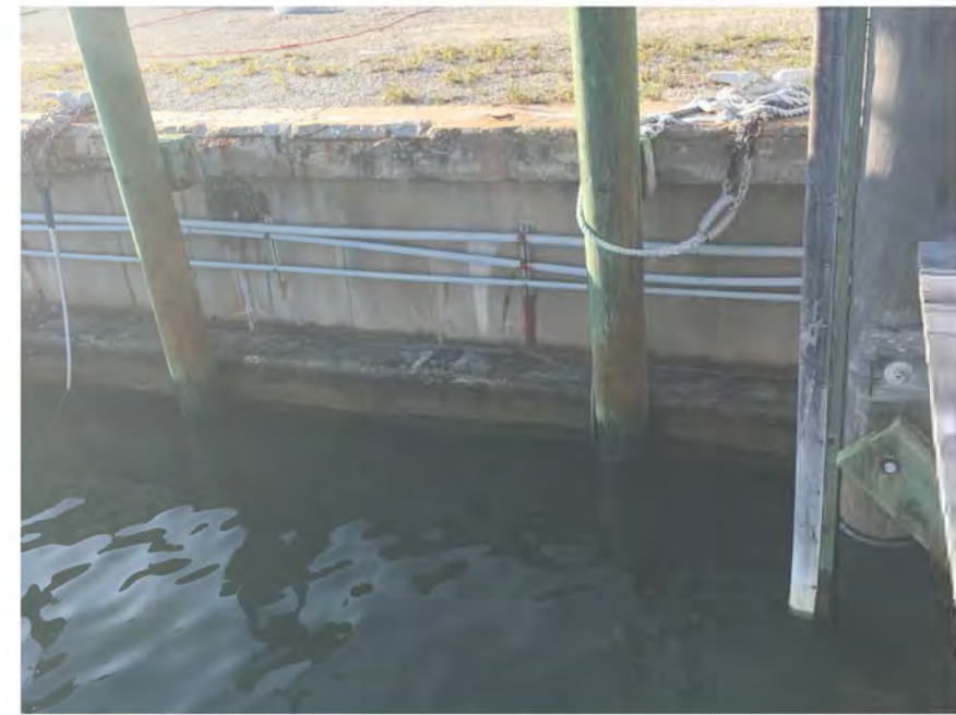
FIGURE 106-A: VIEW OF EXISTING SEAWALL EAST OF DOCK 2
