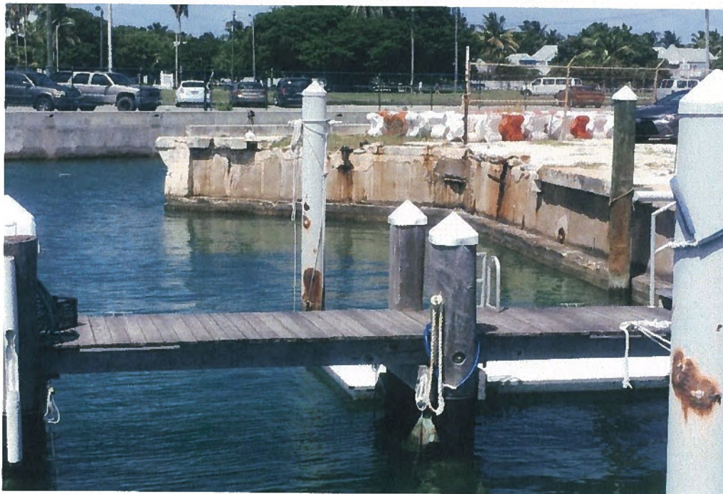
6) East End of Seawall
