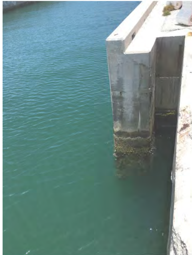
FIGURE 110-A: VIEW OF EXISTING SEAWALL EAST OF TRIANGLE
