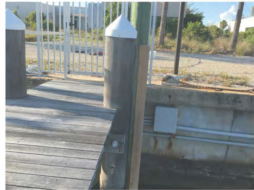
FIGURE 106-B: VIEW OF EXISTING SEAWALL WEST OF DOCK 2
