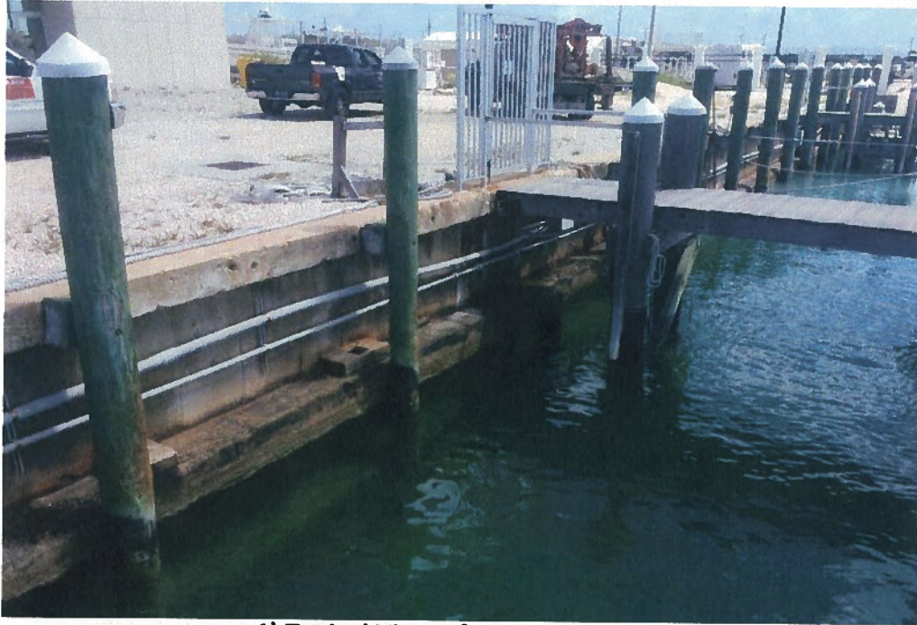
1) Typical View of Existing Seawall
