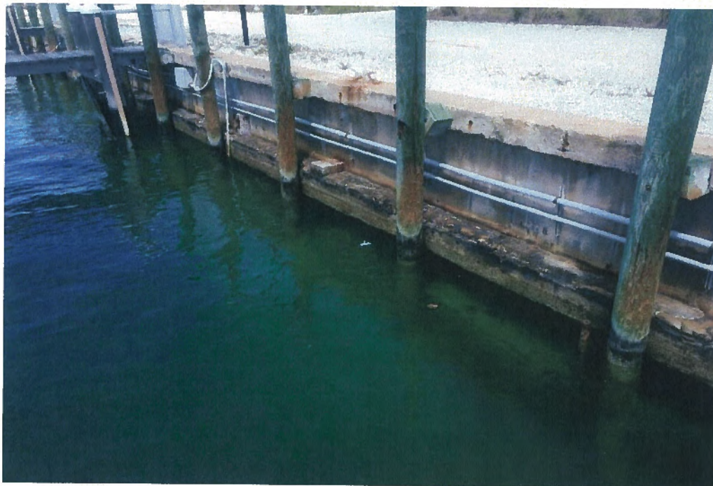
2) Typical View of Existing Seawall
