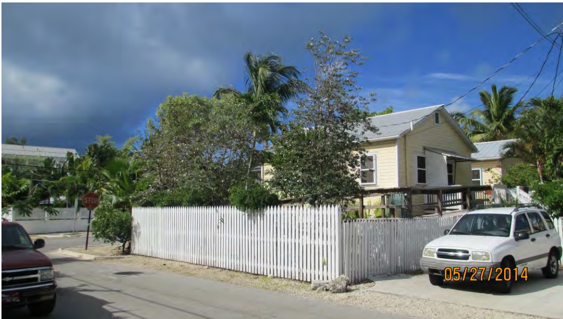
Standing on Dennis St looking southwest toward Venetia, at property. Most of the trees along fence line will not be impacted from demolition and development. Proper tree protection measures will be required. Tree # 77, #77A, and #77B will be removed due to creation of a sidewalk.
