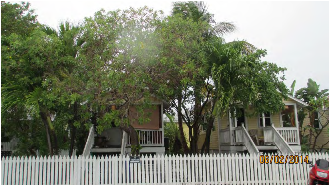
Standing on Venetia looking north into the property. All of these buildings are to be demolished and redeveloped. Trees in this photo include #33, #34, #35, #36, #37, #38, and #39.
