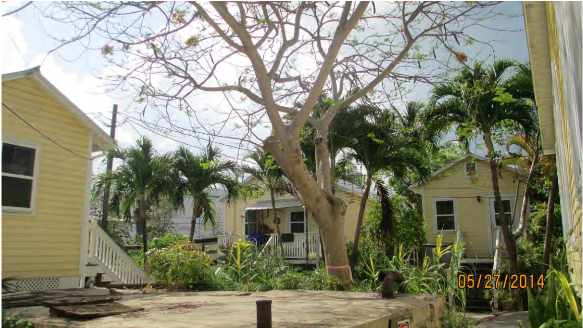
Interior of property looking southeast toward Dennis St. Royal Poinciana to remain and will be protected during demolition and development. Christmas palms in background to be removed.
