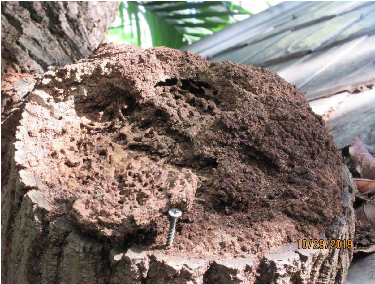
Close up photo of termite frass in old cut.
