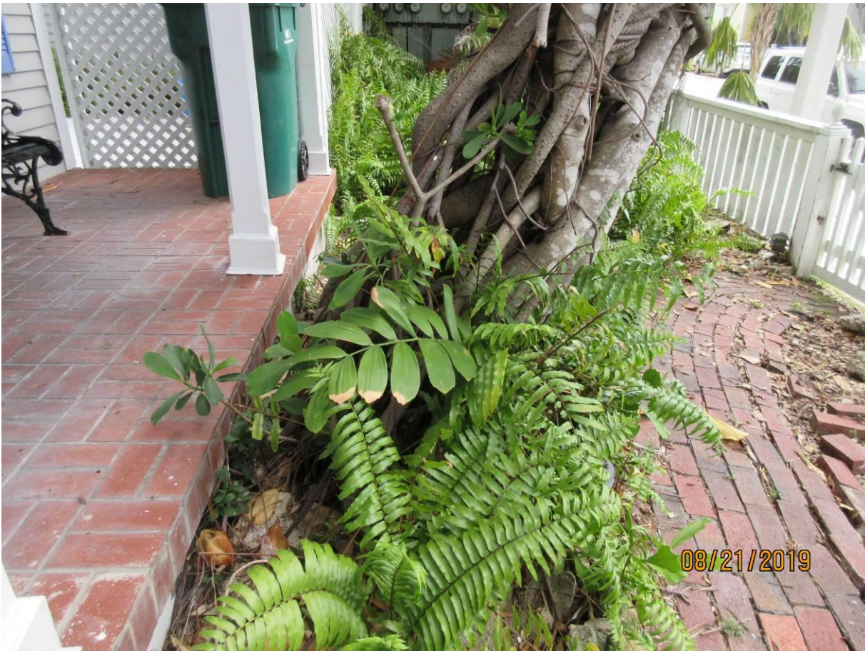
Photo of tree trunk next to structure.
