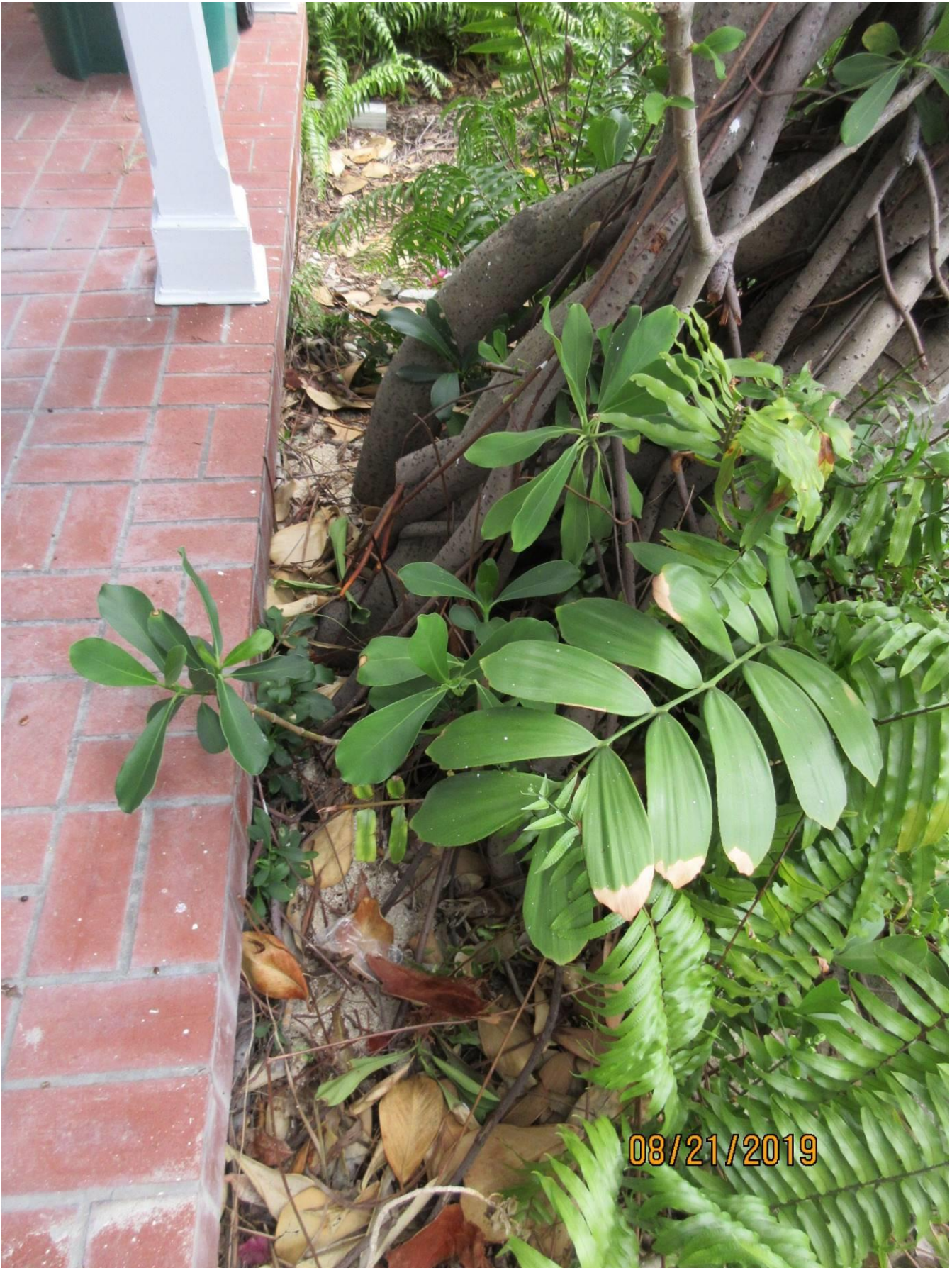
Close up photo of base of tree.
