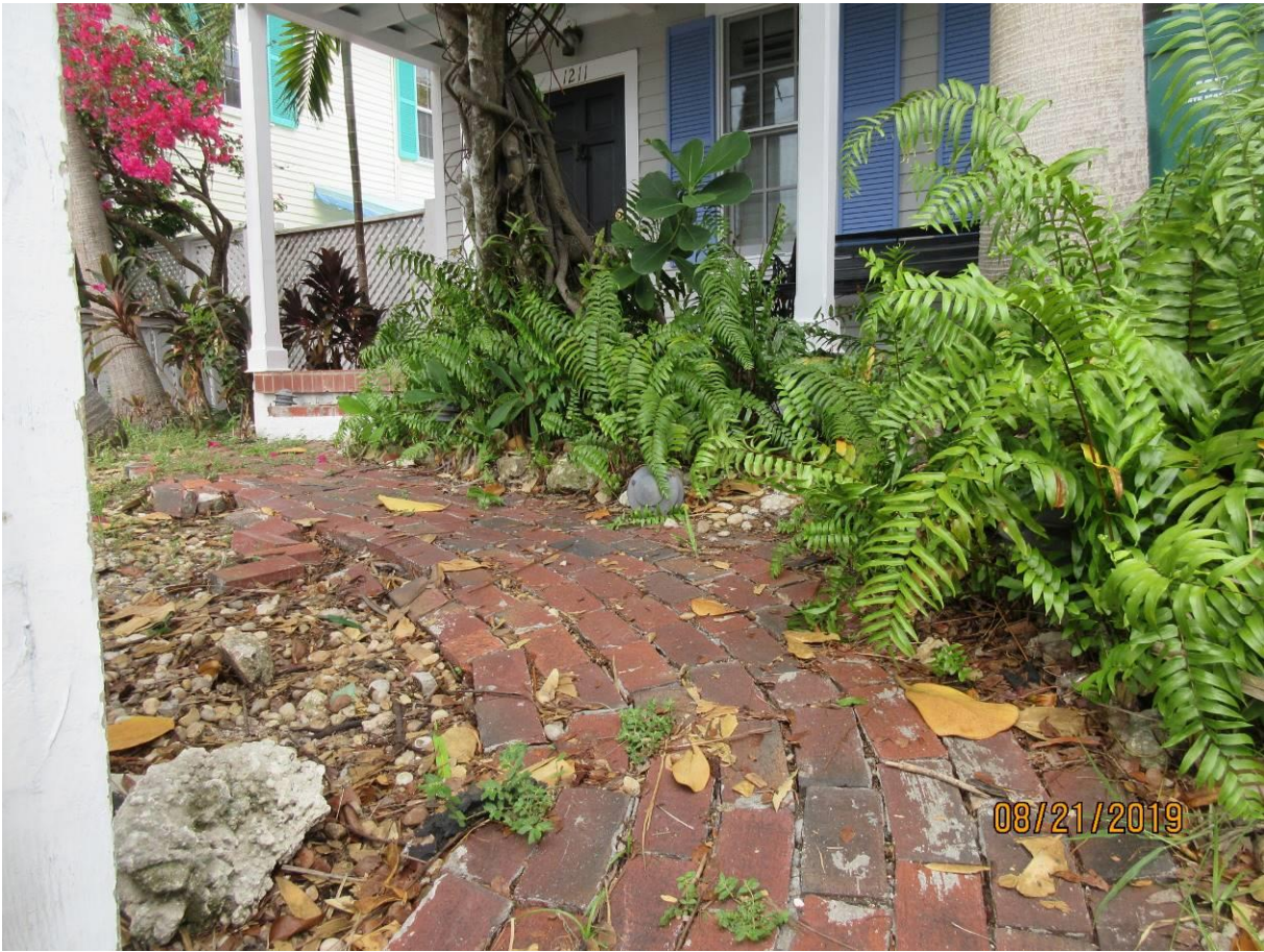
Photo of entrance to house and sidewalk pavers and base of tree.
