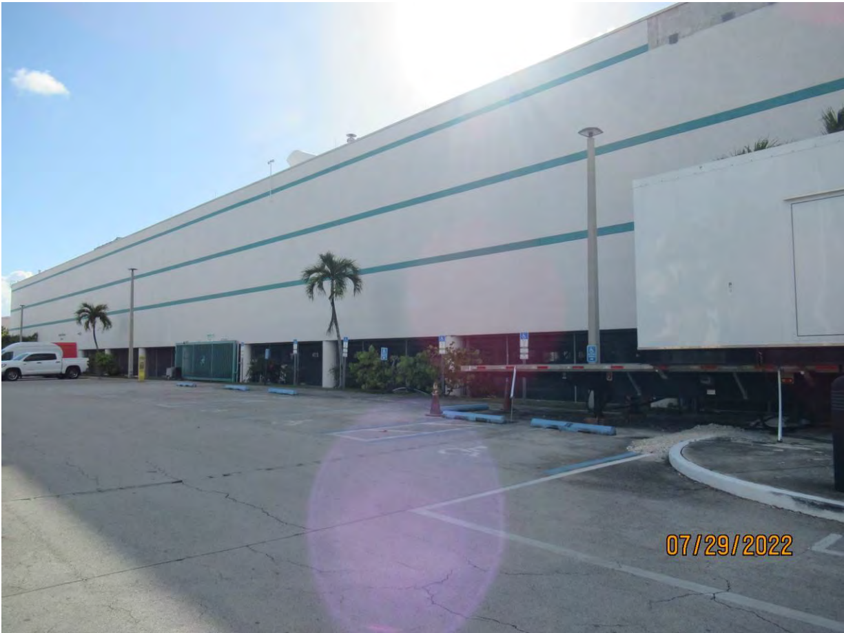
Photo of the proposed generator work area, view 3.
