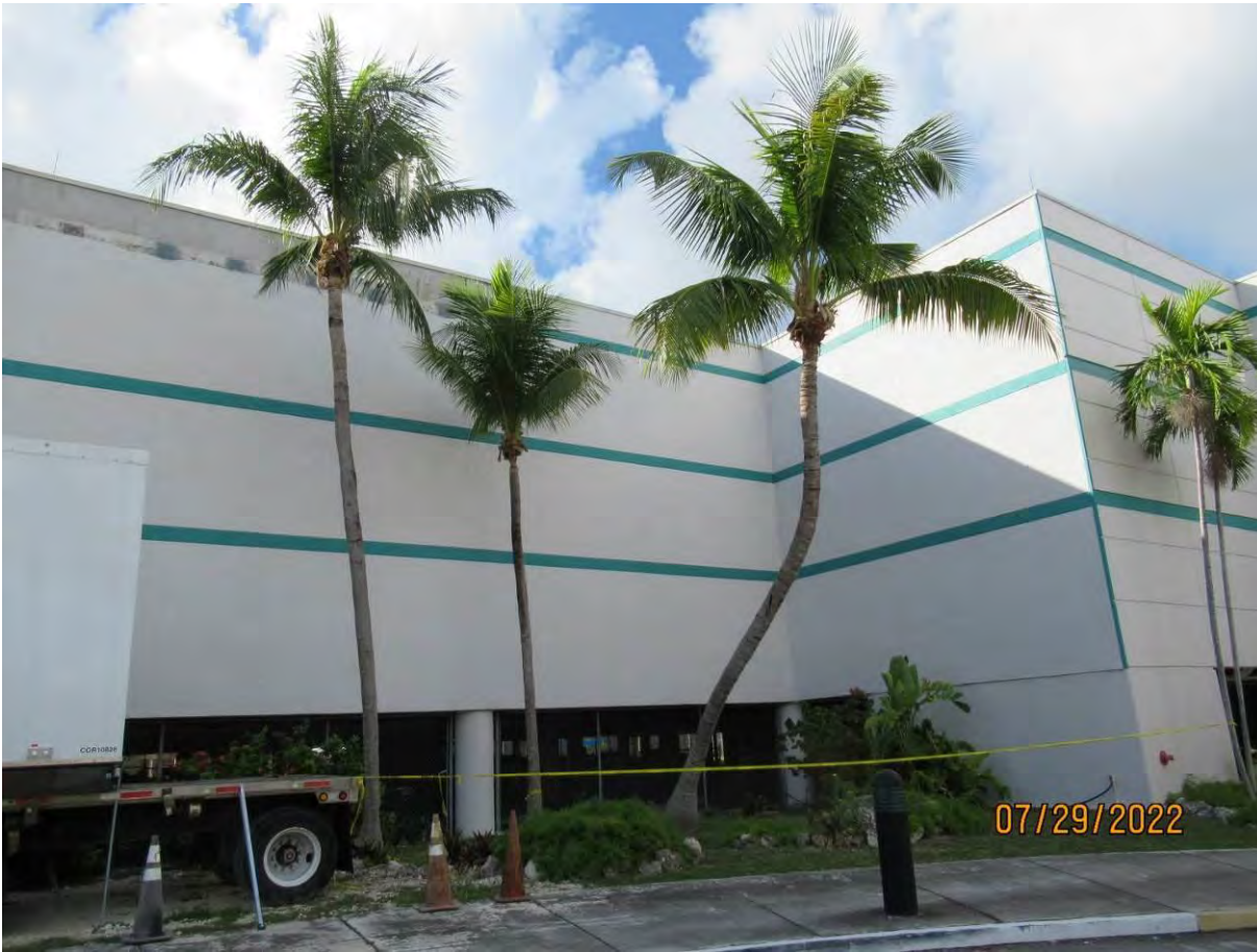
Photo of the proposed generator work area, view 1. Coconut palms are to remain.
