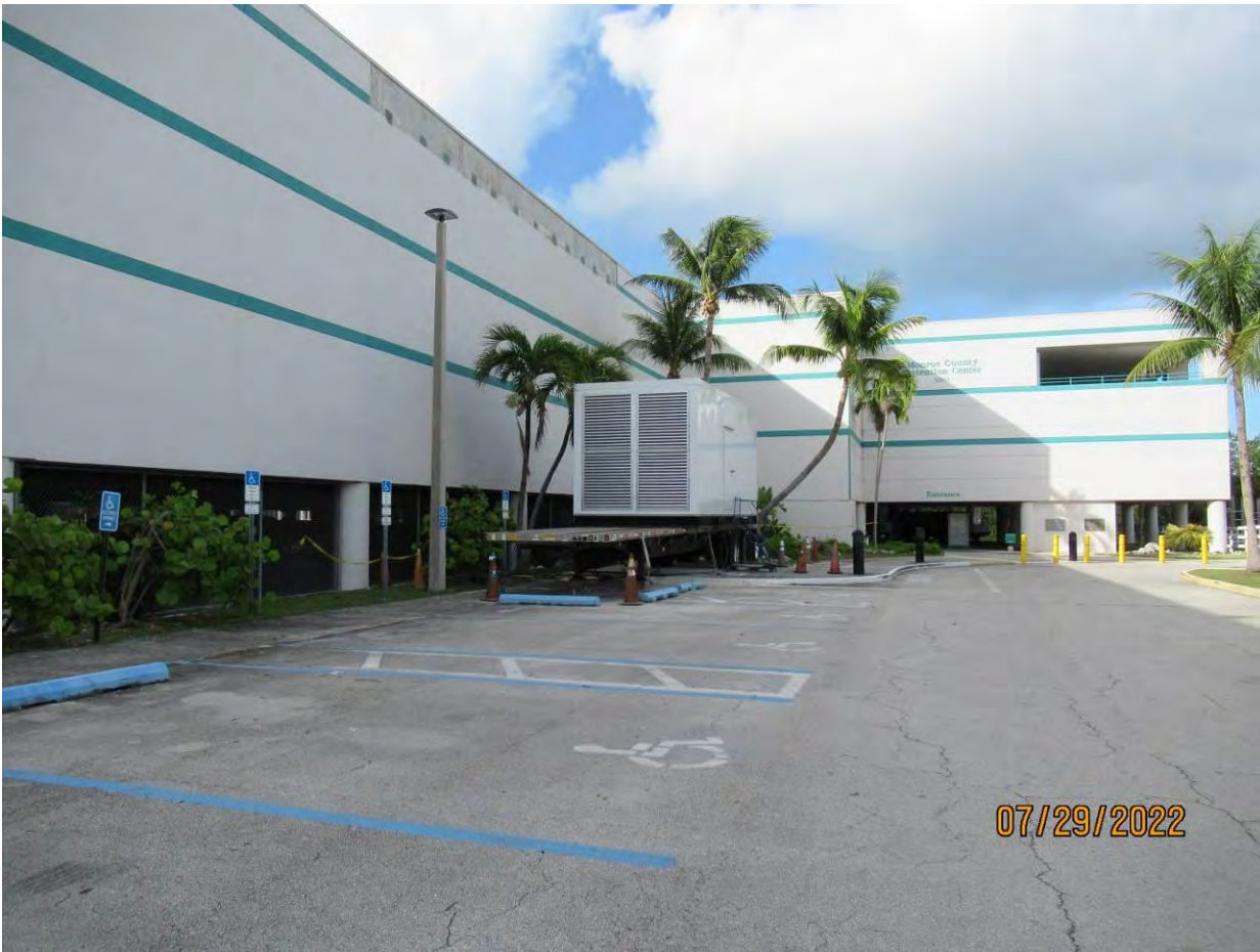
Photo of the proposed generator work area, view 4.
