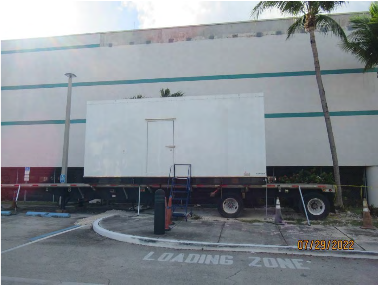
Photo of the proposed generator work area, view 2.
