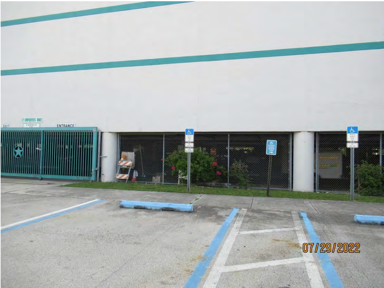
Close up photo of the proposed generator work area, view 3. Shrubs to be removed.
