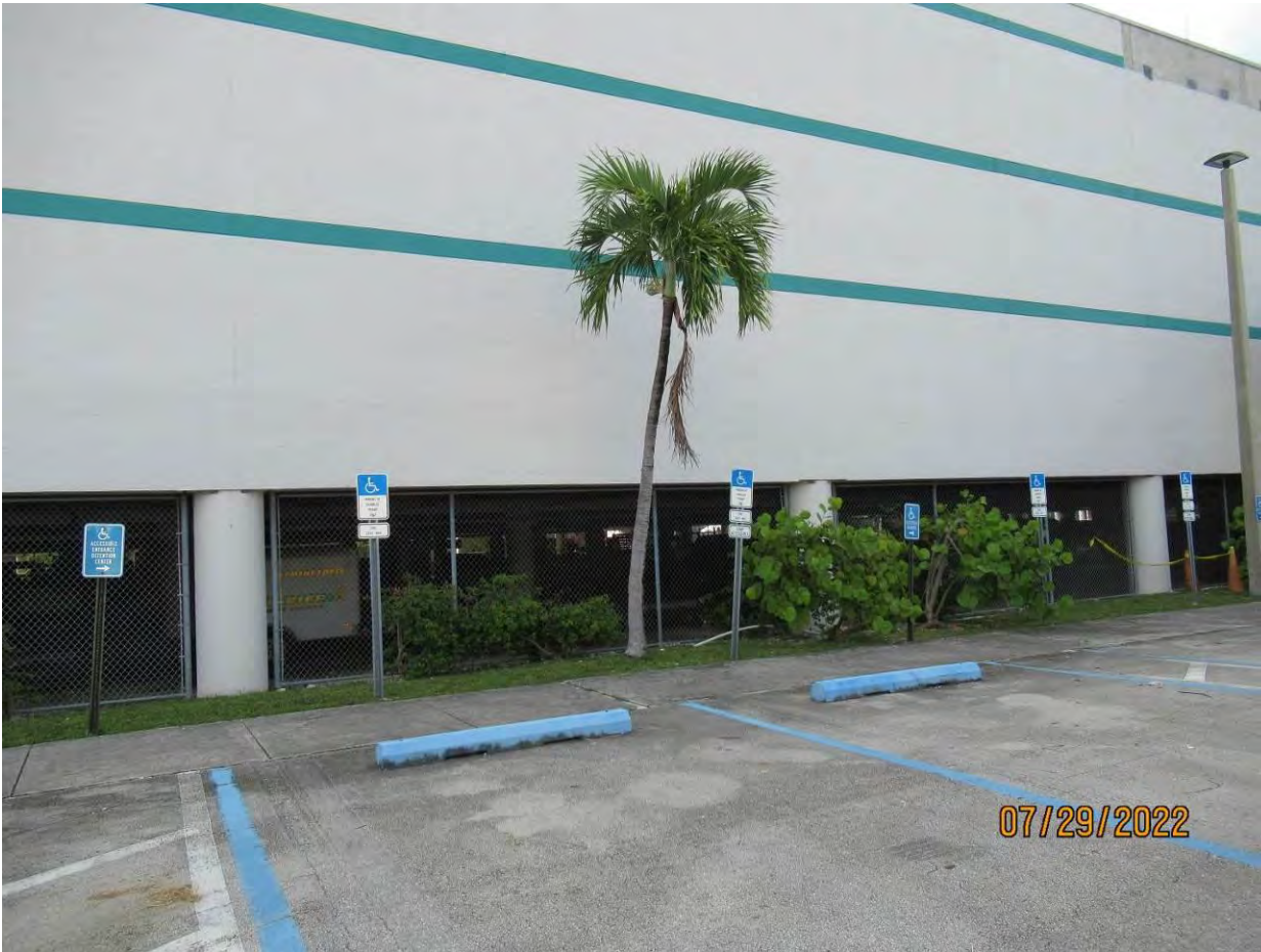
Close up photo of the proposed generator work area, view 2. Christmas palm to be transplanted and shrubs to be removed.
