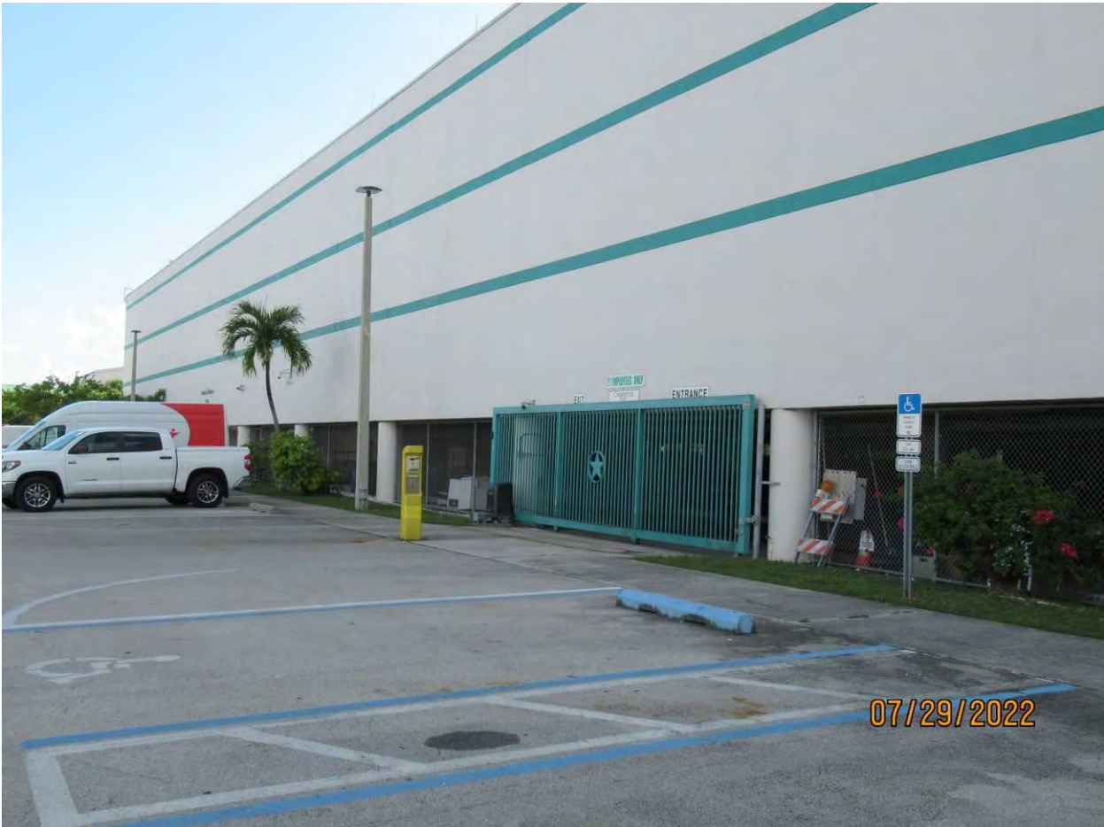
Photo of the proposed generator work area, view 5. New parking lot island with a tree to be created in this area.
