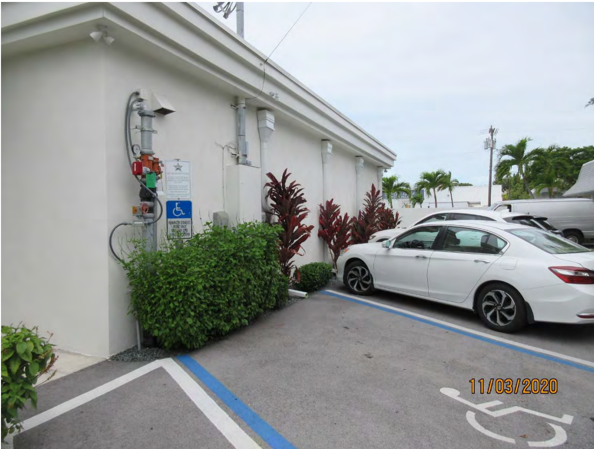
Photo showing rear of the building.
