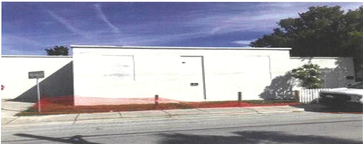
Band Room & Industrial Arts Building (2020)
