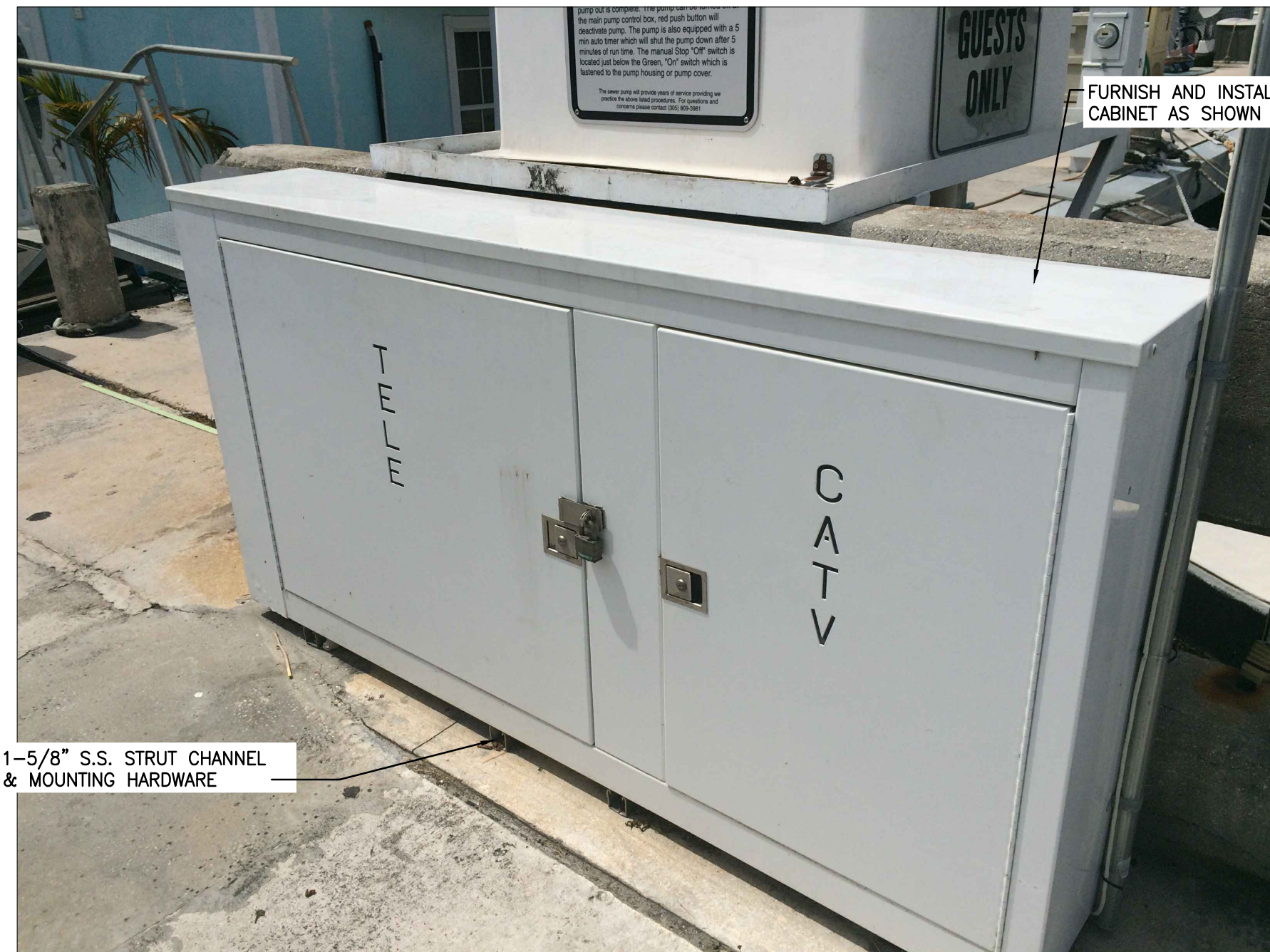
TELE/CATV CABINET DETAIL NO SCALE
