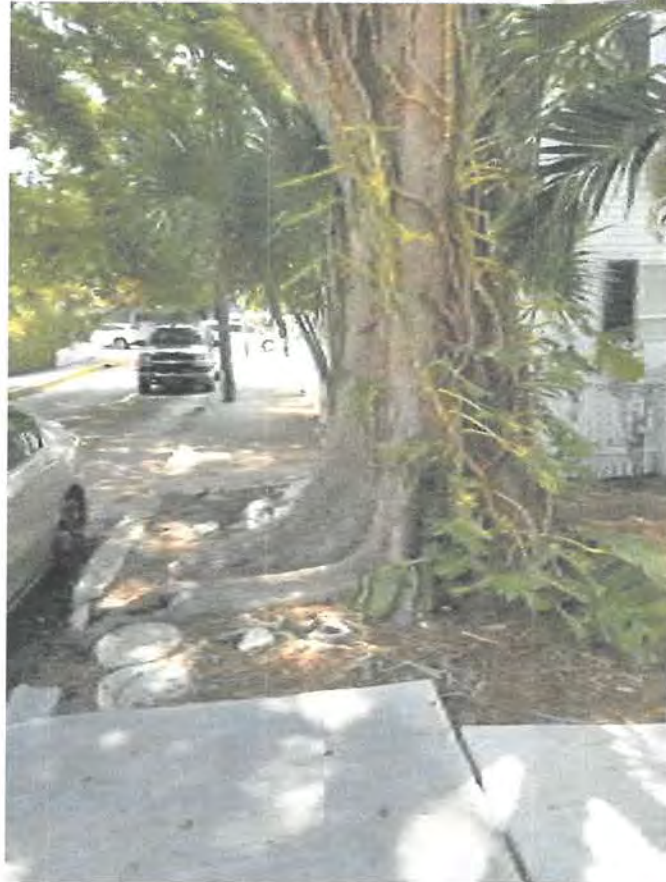
Photo 2. View of tree from north. Sidewalk is missing, adjacent pavers and curb broken.
