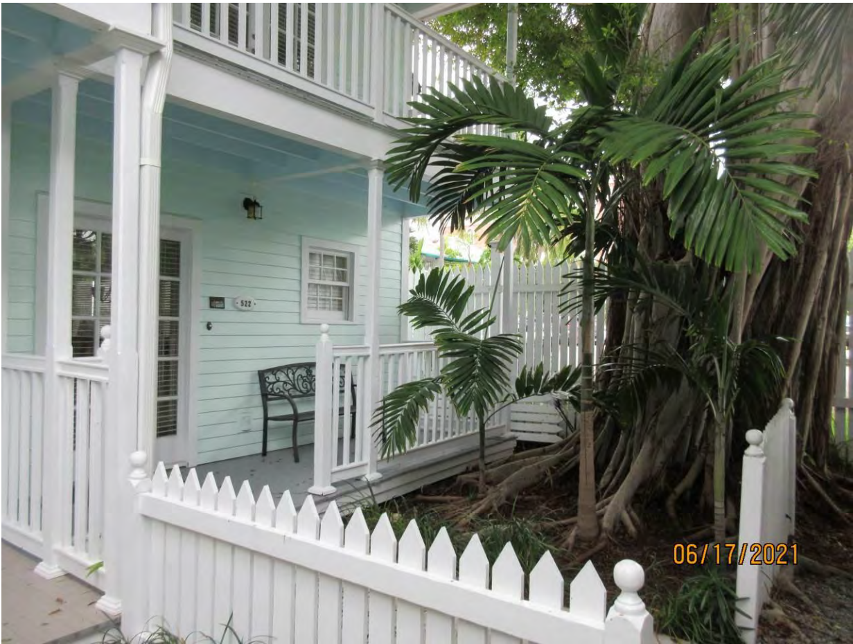
Photo showing location of base of tree and trunk and structure.
