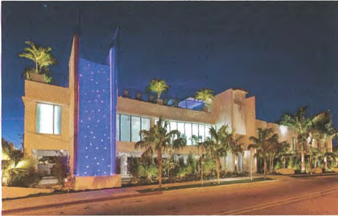
SIMONTON STREET ELEVATION AT NIGHT
