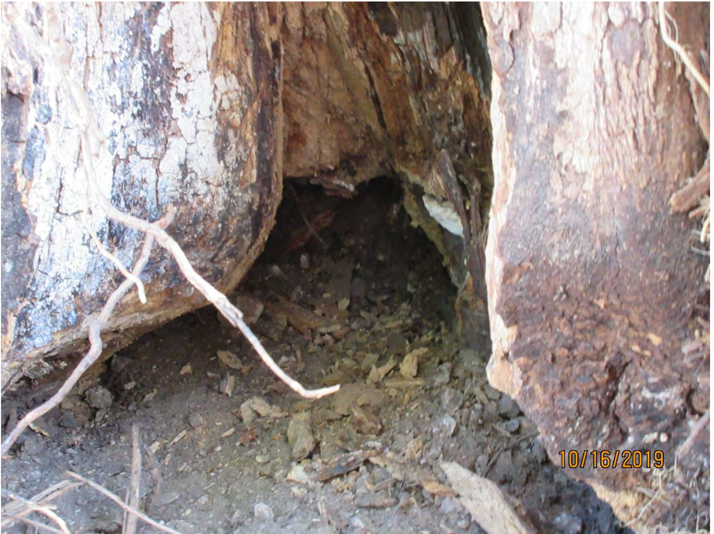
Close up photo of hole/decay area, view 2.
