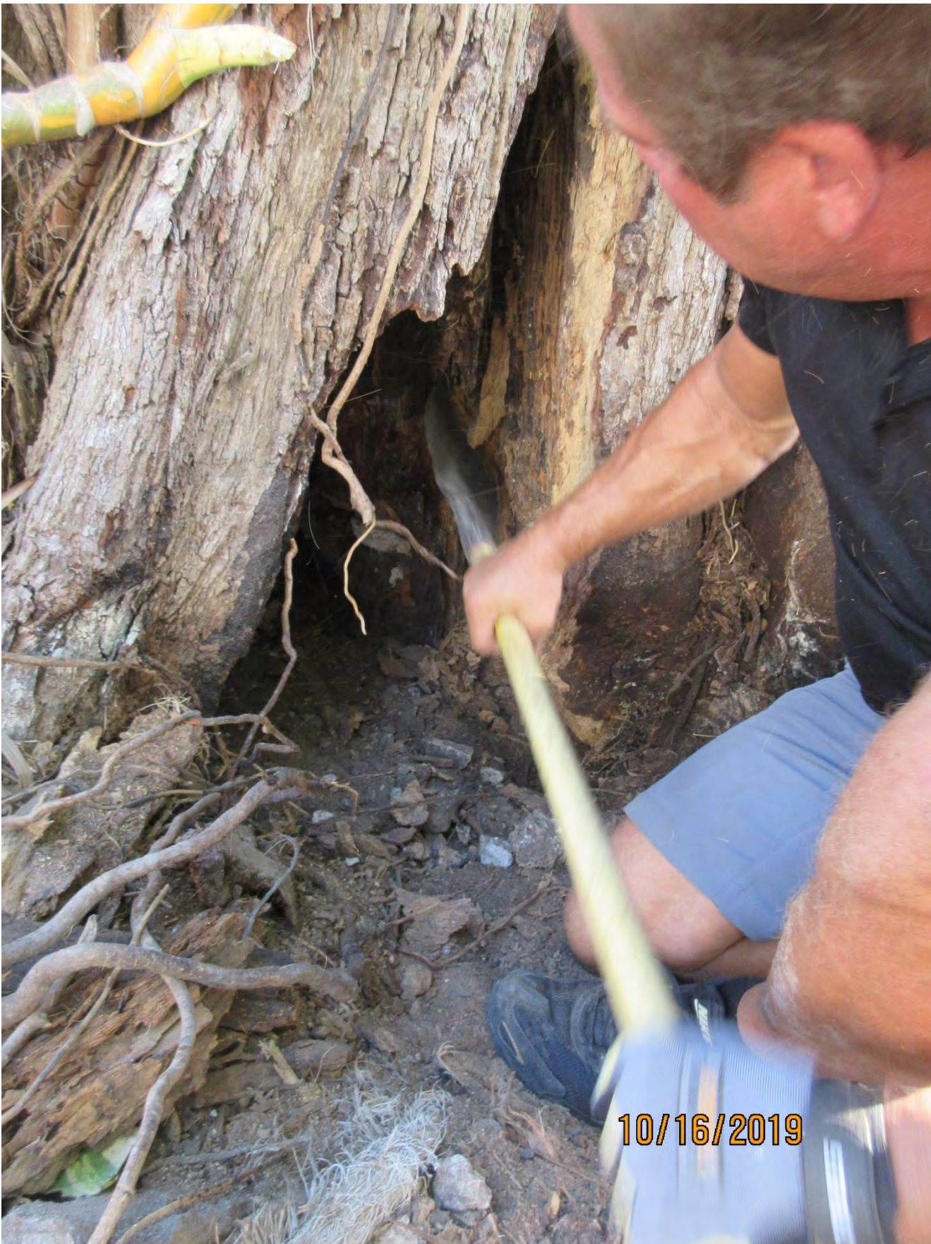
Photo showing the interior decay. Shovel would tap the wood and it would fall off easily.
