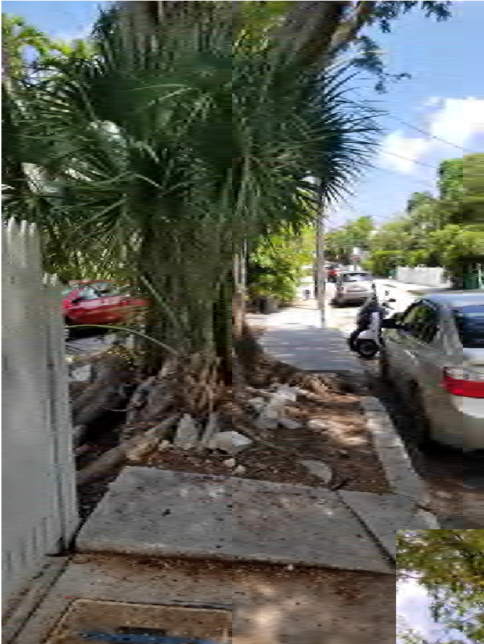
Photo 3. View of base of tree from the south.
