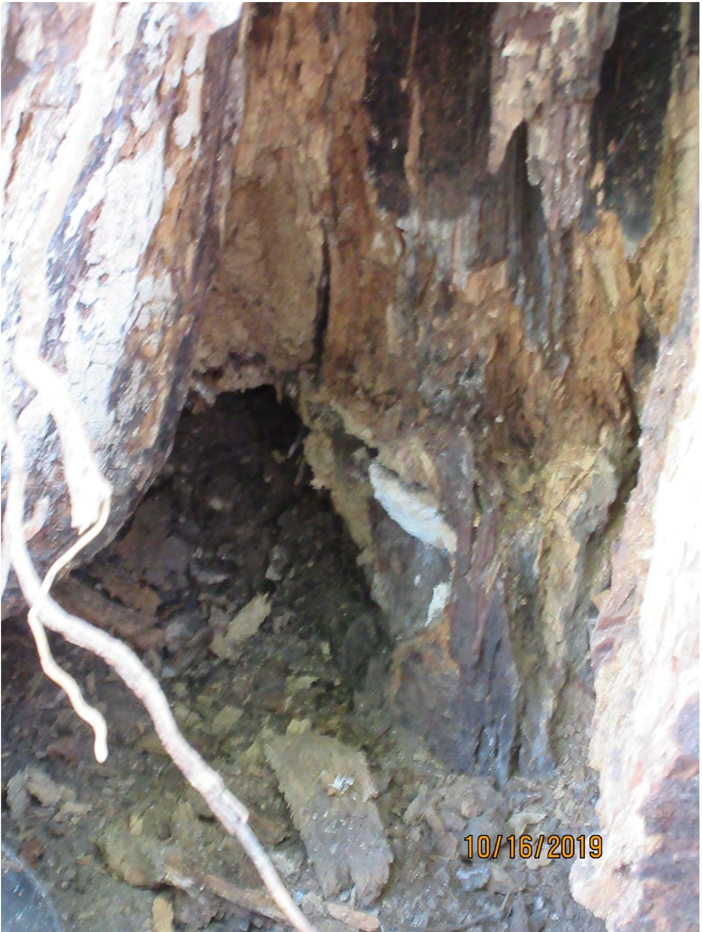
Close up photo of hole/decay area, view 1.
