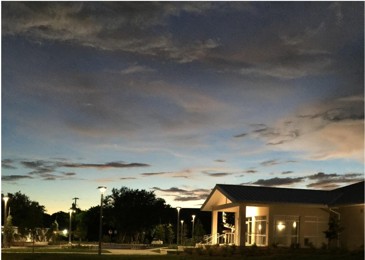
Exterior Lighting at Marathon City Hall
