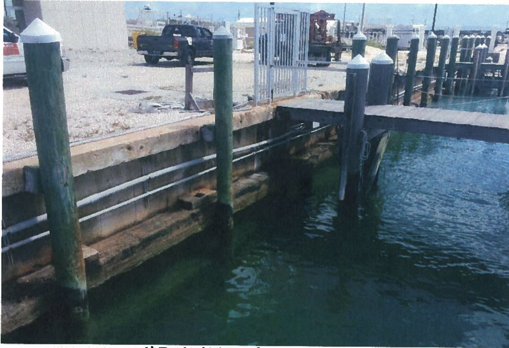
1) Typical View of Existing Seawall
