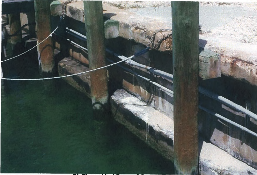
5) Close-Up View of Seawall Front
