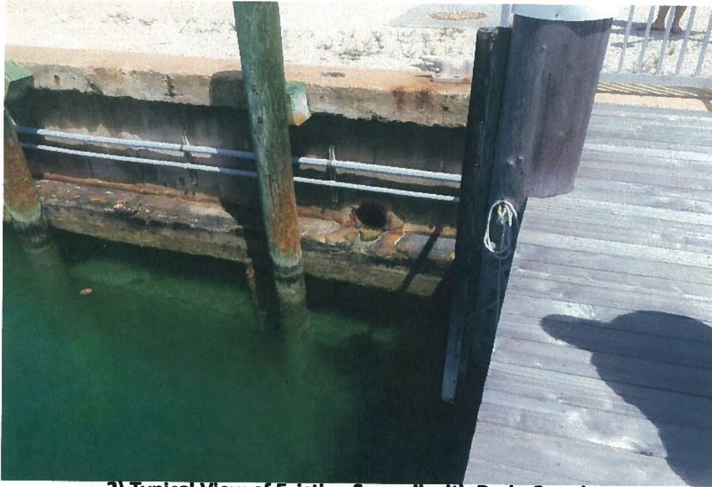
3) Typical View of Existing Seawall with Drain Crossing
