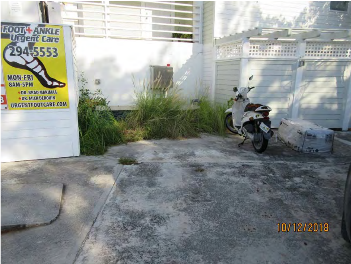
Front of existing building
