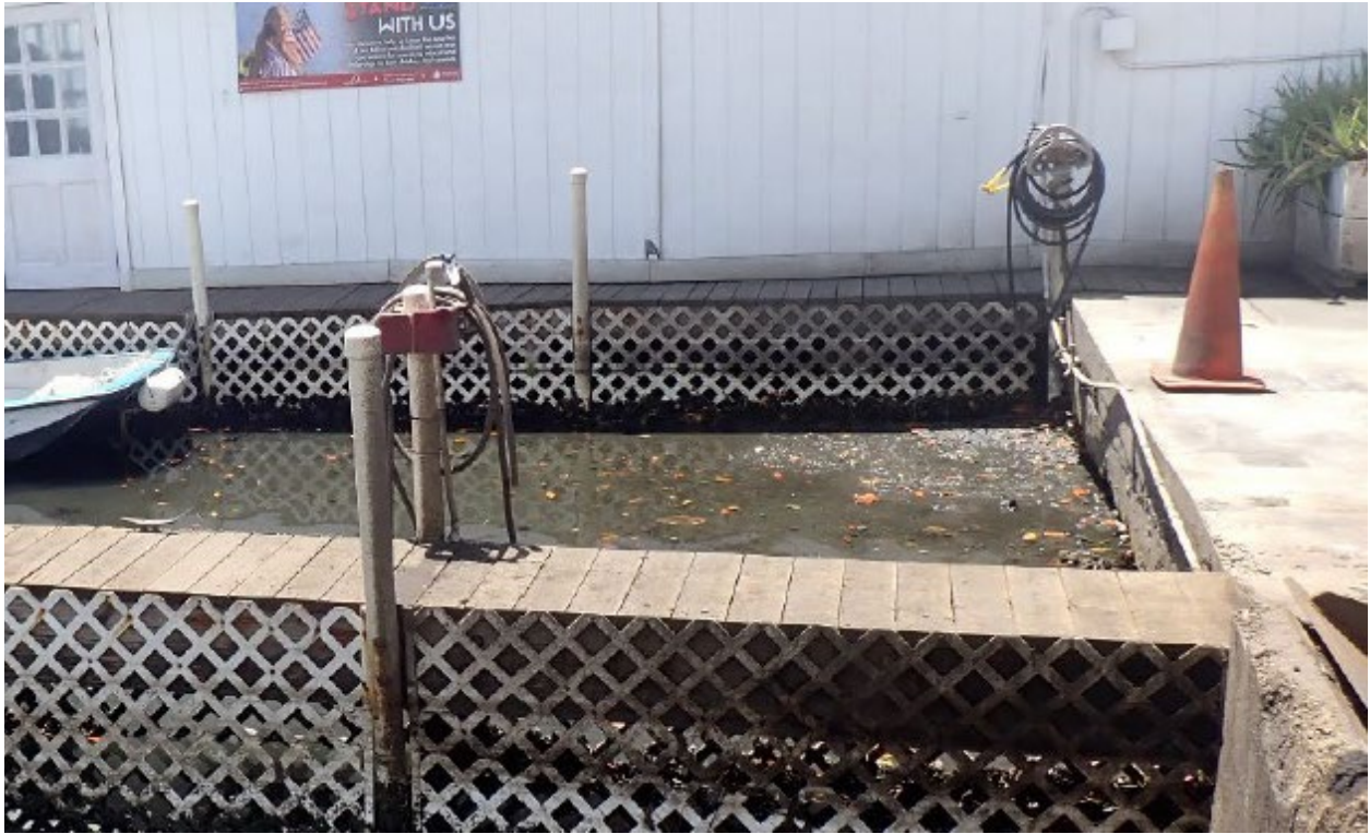
Photos along the marina's seawall/bulkhead show that sediment has accumulated up to the water line.
