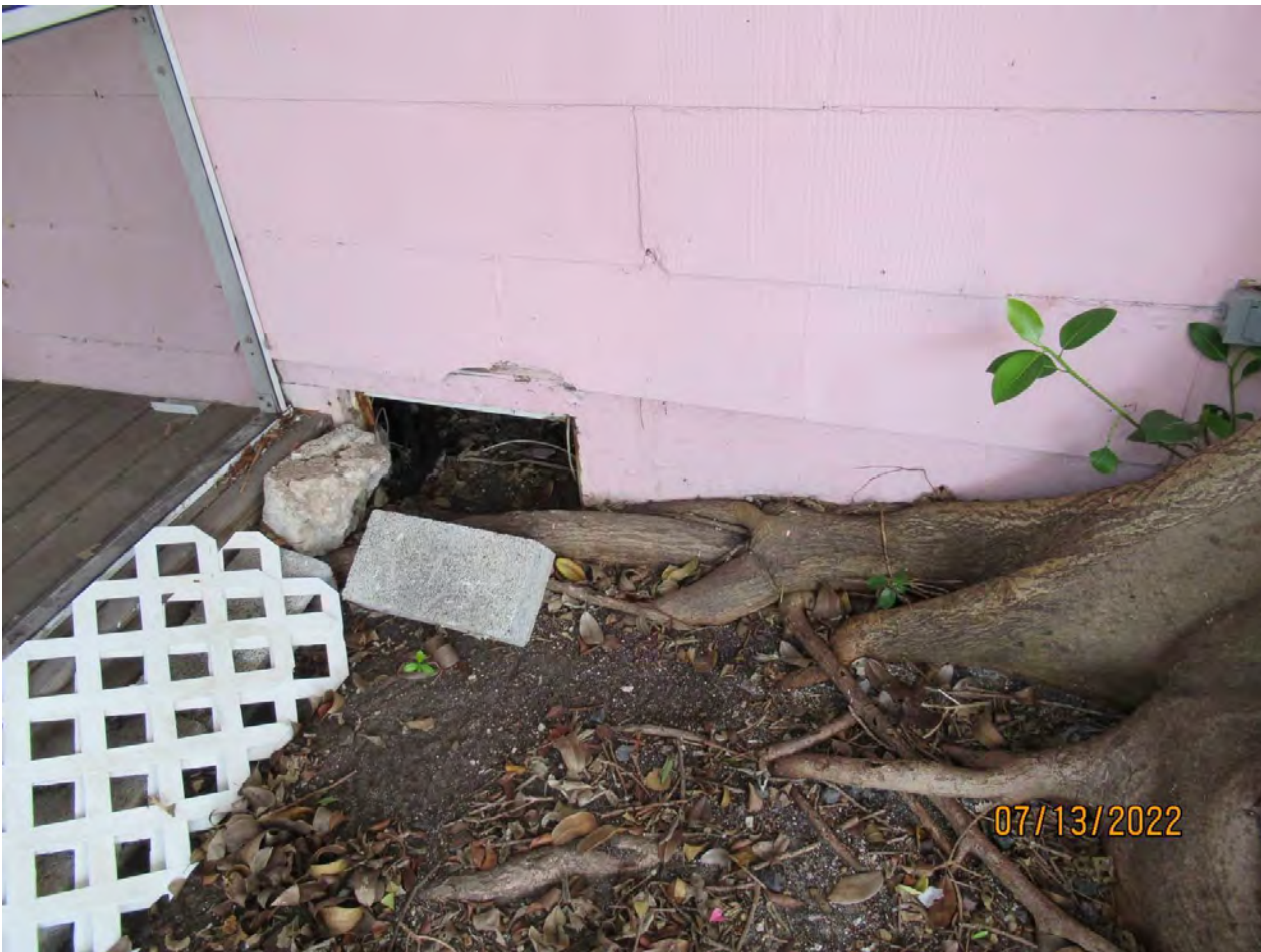
Photo of a main tree root along foundation pier, view 2.
