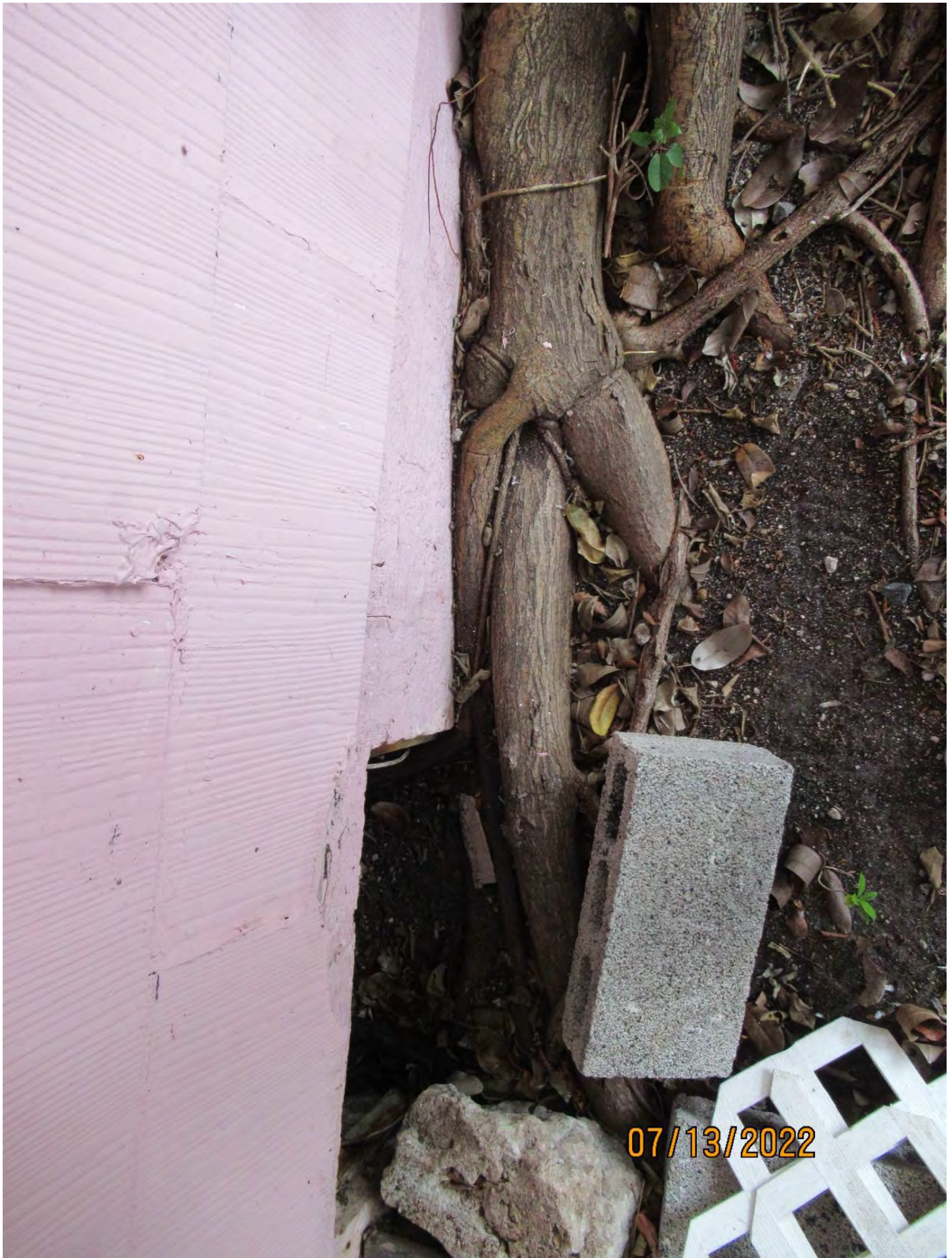
Photo of a main tree root along foundation pier, view 1.
