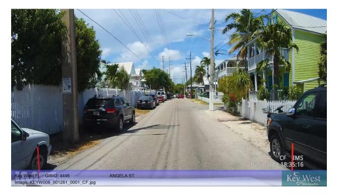
Angela Street from Chapman Lane to Thomas Street (GISID 4446, PCI = 71) – Rated as Very Good, this road displays minor amounts of longitudinal cracking and edge cracking. The surface is non-weathered, and the base is still strong. This street is an example of a candidate for preventative maintenance and light weight surface treatments to extend the life of a roadway.
