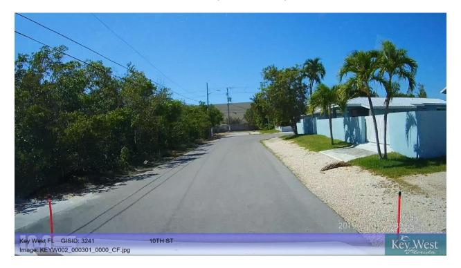
**10**<sup>th</sup> **Street from Patterson Avenue to Fogarty Avenue (GISID 3241, PCI = 92)** – Rated as Excellent, displaying little to no surface distresses. The ride is smooth and the surface is non-weathered and the base is strong. In a couple of years, this street segment would be an ideal candidate for routine maintenance activities such as crack sealant service.
