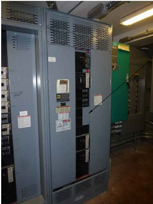
2000A 277/480V PANEL MAIN ELECTRICAL ROOM
