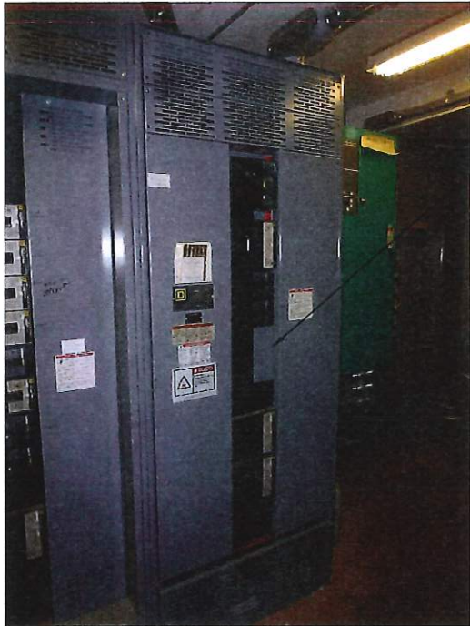
2000A 277/480V PANEL MAIN ELECTRICAL ROOM
