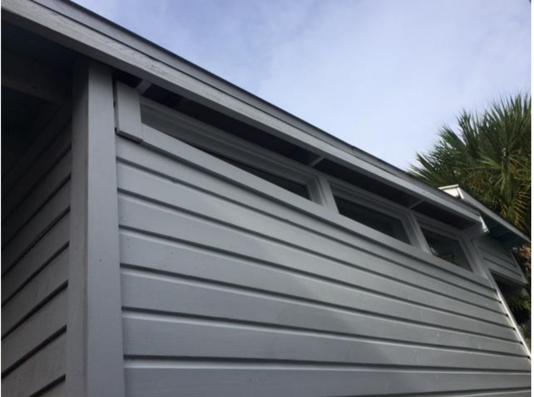
Close-up of side addition. The side wall and window will remain. A new gable roof will be constructed on top.
