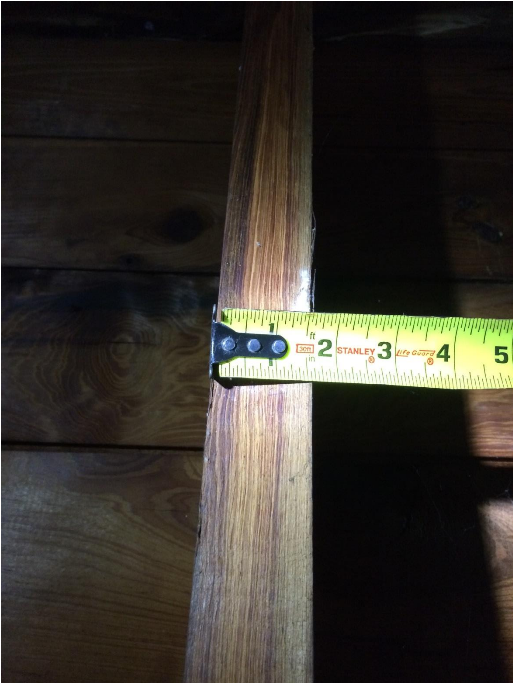
Photo: Existing Conditions; New 1-1/2" Nominal Lumber
