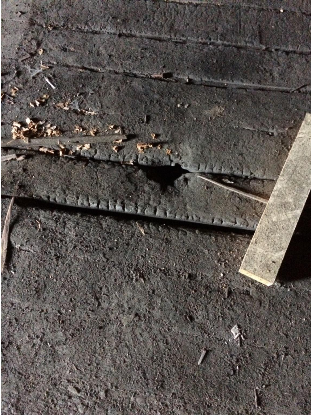
Photo: Existing Conditions; Charred Attic Flooring
