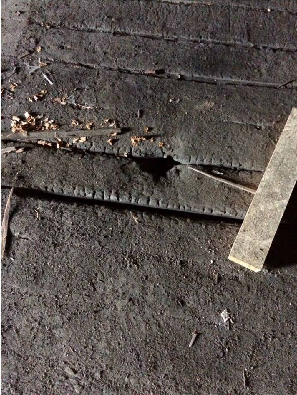
Photo: Existing Conditions; Charred Attic Flooring
