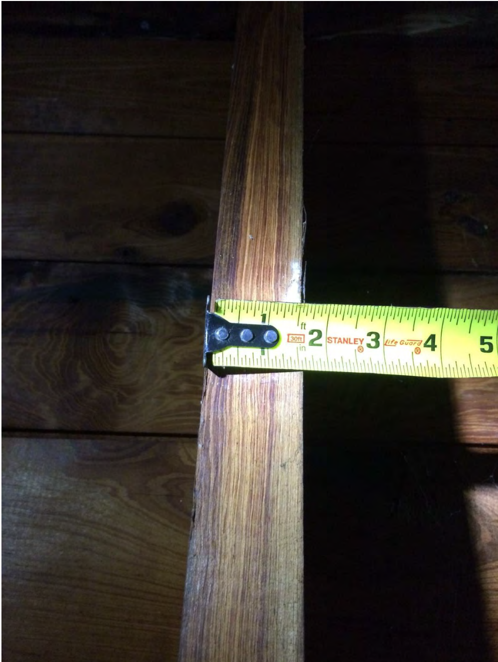
Photo: Existing Conditions; New 1-1/2" Nominal Lumber
