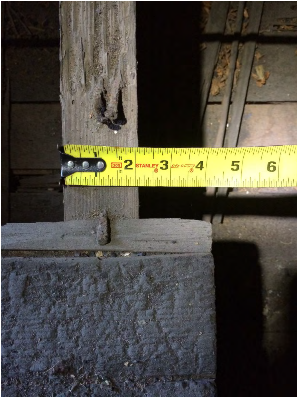
Photo: Existing Conditions; Original 2" Lumber
