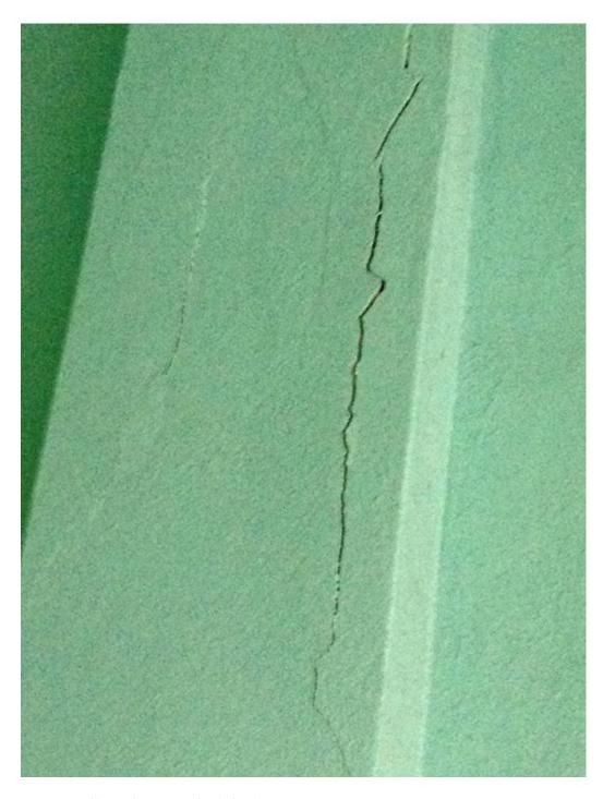
Note cracking along steel reinforcing
