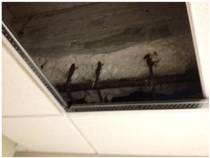
Note missing 6" plus of concrete with exposed severely rusted rebar
