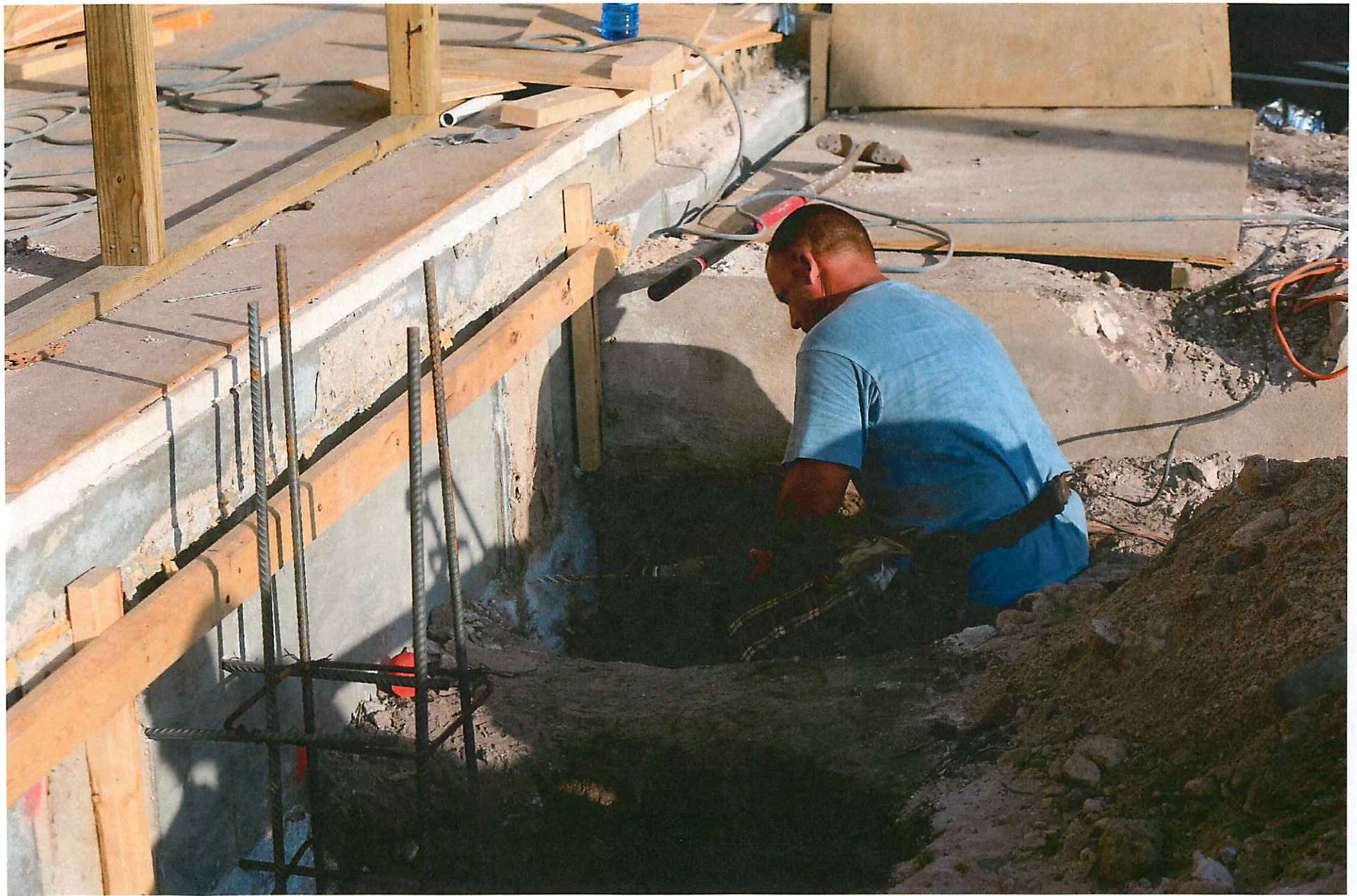
New foundation piers to carry increased loads old foundation piers were set on top soil
