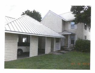
Roof attic areas meet code requirements for ventilation. Some vinyl soffits were loose and require fastening. Vinyl vented soffits are clipped to fascia and wall truss tails, a fair amount of vinyl fascia is dislodge or damaged.
