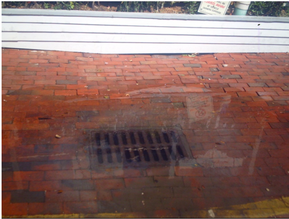
Inlet behind the wall not draining, notice the sinking of the brick. (Low to mid – tide)
