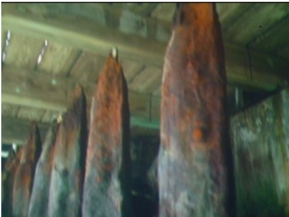
Corroded Steel to be Removed
