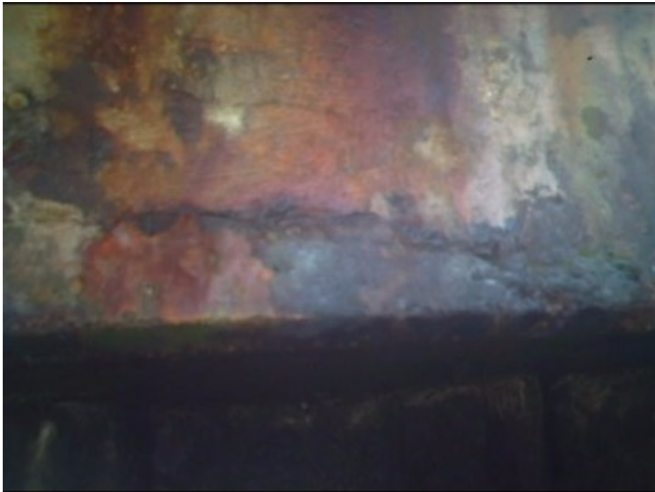
Cracks in the Sea Wall Cap
