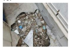
**Location:** Exterior Rear **System:** Exterior **Condition:** Washed Out Area Of Grading **Explanation:** A section of grading is not level to a point at which it may pose a safety hazard.
