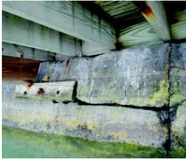
Photo 14: Cracking from Sta 52' C thru Sta 58' C
