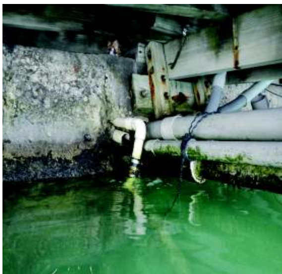
Photo 29: Utility penetrations at Sta 15' E
