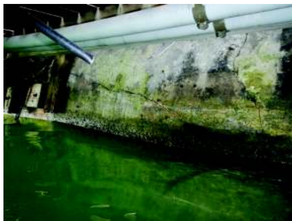
Photo 18: Cracking in wall at Sta 133' C
