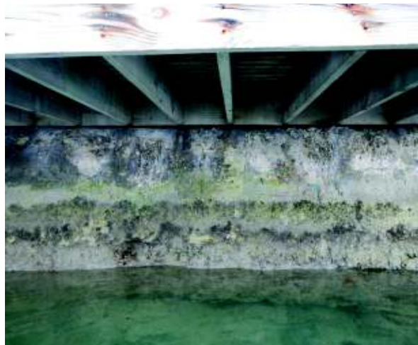
Photo 26: Condition of restaurant deck overhang
