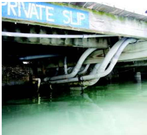
Photo 30: Utility penetrations at Sta 15' E
