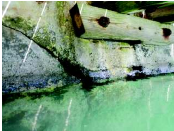
Photo 16: Cracking in wall at Sta 110' C
