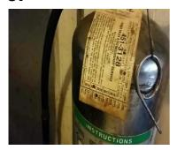
**Location:** Kitchen **System:** Interior **Condition:** Expired Fire Extinguishing
