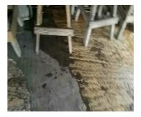
**Location:** Lounge **System:** Interior **Condition:** Trip hazard in floor surface **Explanation:** The floor surface has an abrupt change in height where different floor finishes abut. This condition has a variation that is sufficiently great as to present a potential trip hazard.
