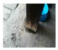
**Location:** Outdoor Dining **System:** Structure **Condition:** Rot in wood column(s) **Explanation:** Support columns are crucial to providing proper transfer of building loads to the footings. Areas of wood rot and deterioration are observed. Selective probing indicates loss of fiber strength and integrity. The current and future ability of the column(s) to bear their intended load is suspect.
