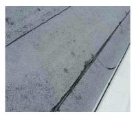
Location: CBS Bldg Roof System: Roof Condition: Bubbled Roll Roofing
