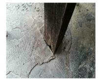
**Location:** Outdoor Dining **System:** Structure **Condition:** Rot in wood column(s) **Explanation:** Support columns are crucial to providing proper transfer of building loads to the footings. Areas of wood rot and deterioration are observed. Selective probing indicates loss of fiber strength and integrity. The current and future ability of the column(s) to bear their intended load is suspect.
