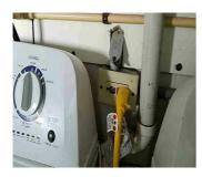
**Location:** Kitchen **System:** Electrical **Condition:** Electrical outlet is damaged **Explanation:** An electrical outlet is observed to be damaged. The usual cause is due to impact or other forms of mechanical action to fracture the insulating body of the outlet.
