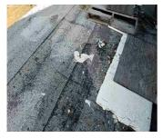
**Location:** Exterior Left **System:** Roof **Condition:** Asphalt roll roofing is old **Explanation:** The shingle roof surface is displaying indicators that the protective roof covering is at or near the end of its service life.
