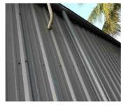
Location: Exterior Right System: Exterior Condition: Unsealed AC Condensate
