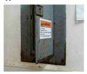
Location: Kitchen System: Electrical Condition: Evidence of water at electrical distribution or sub panel.
