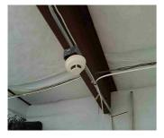
**Location:** Office **System:** Electrical **Condition:** Detector [smoke fire or CO] is loose **Explanation:** A smoke fire or carbon monoxide detector is observed to be not adequately secured at its present location.
