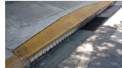
Type 6 Inlet Filter
