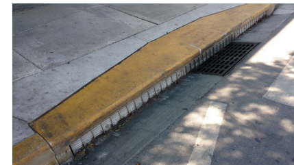
Type 6 Inlet Filter
