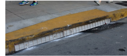
Type 5 Inlet Filter
