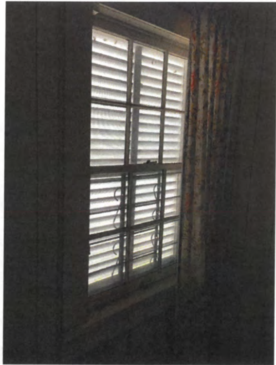
Existing bedroom non-historic 6 over 6 window to be removed for proposed wood French doors.
