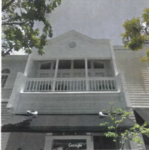
CLADDING EXISTING SLIM COLUMNS TO THICKER POSTS
