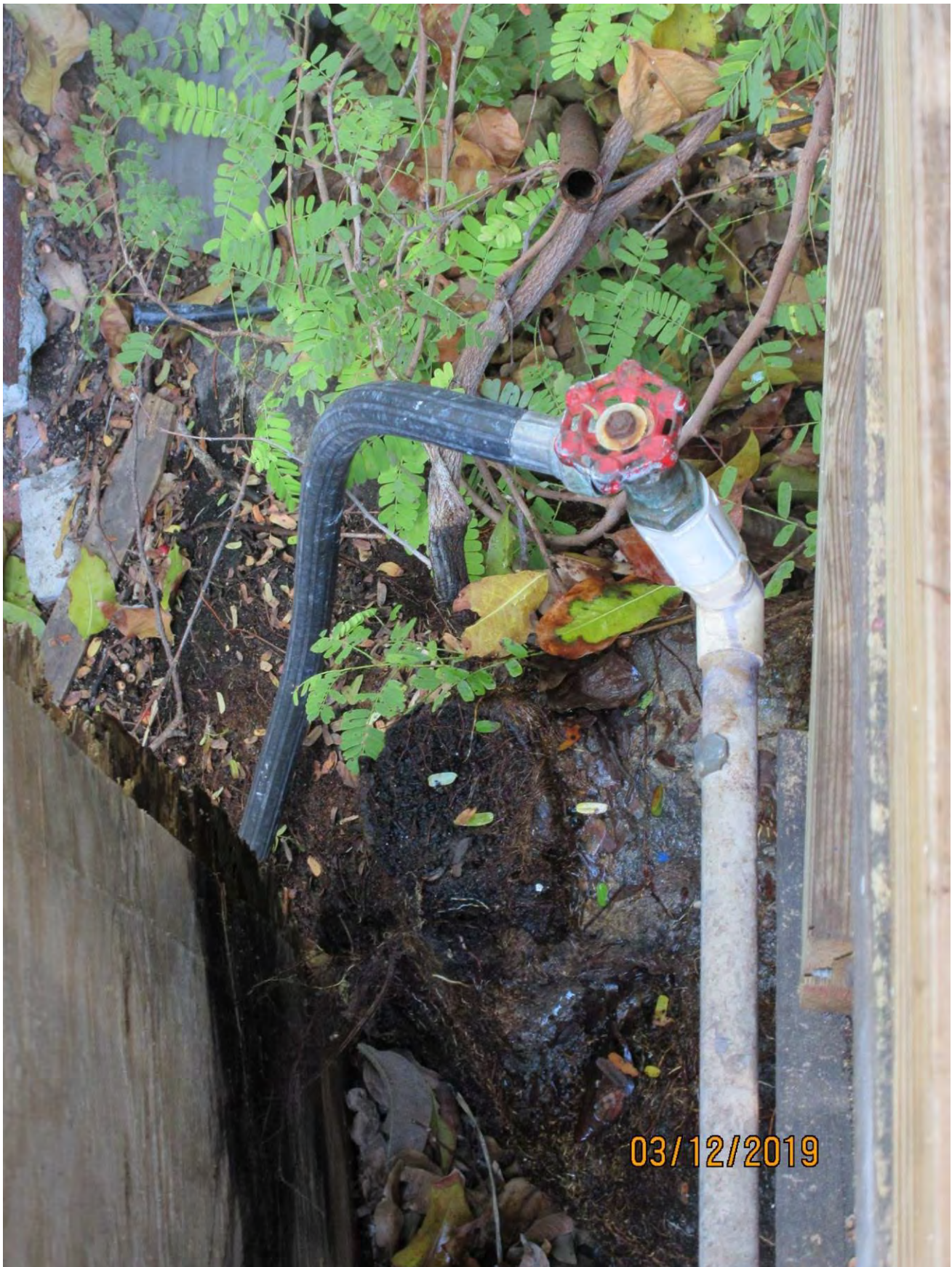
Leaking spigot on neighboring property next to tree (photo taken looking over the fence).
