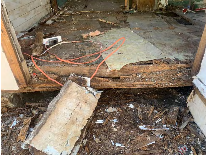
DETERIORATED REAR SILL BEAM AT SAWTOOTH
