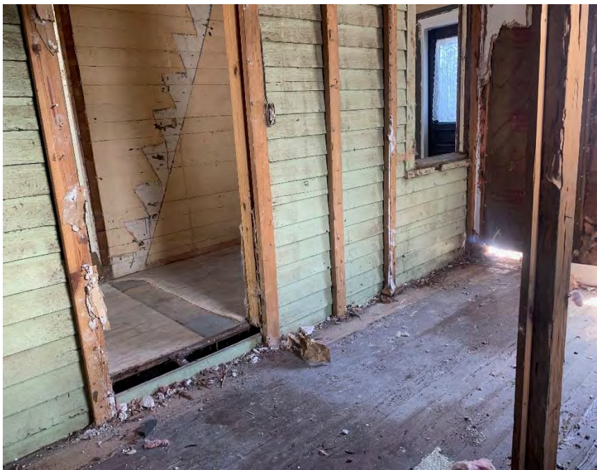
WEST WALL OF ORIGINAL HISTORIC STRUCTURE TO BE EXPOSED WITH REMOVAL OF WEST ADDITIONS
