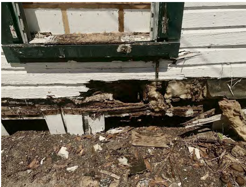
DETERIORATED FRONT SILL BEAM AT SIDE ADDITION
