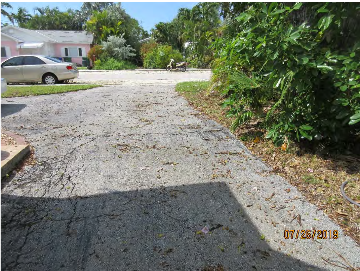
Photo of driveway showing root damage, view 1.
