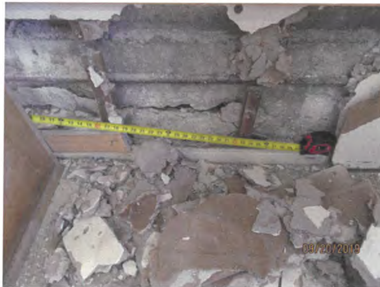
Cracked Foundation Stem Wall Opposite Royal Poinciana
