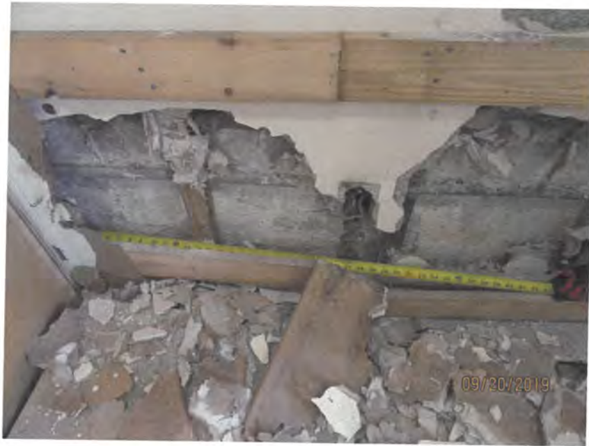
Cracked Foundation Stem Wall Opposite Mahogany
